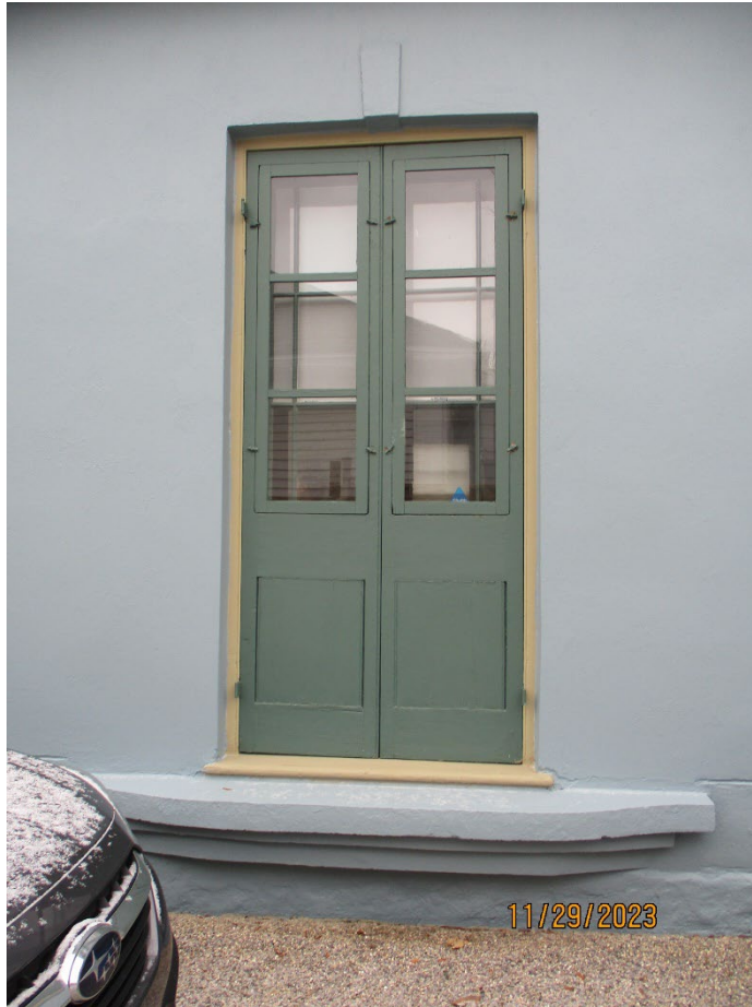
Image 29: Photograph of the painted wood French doors and painted wood storm doors in the opening of the west façade, sill as an indication of the former verandah of Carfrae Cottage (2023).
