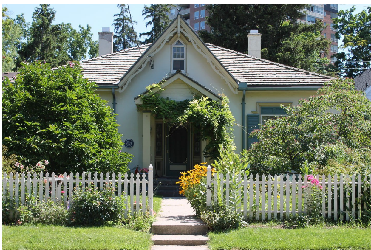
Image 2: Photograph of Carfrae Cottage on July 21, 2015.
