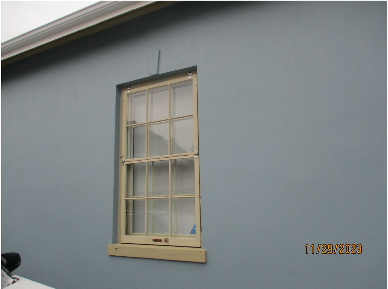
Image 31: Photograph of the painted wood six-over-six shingle hung wood window on west façade (2023).
