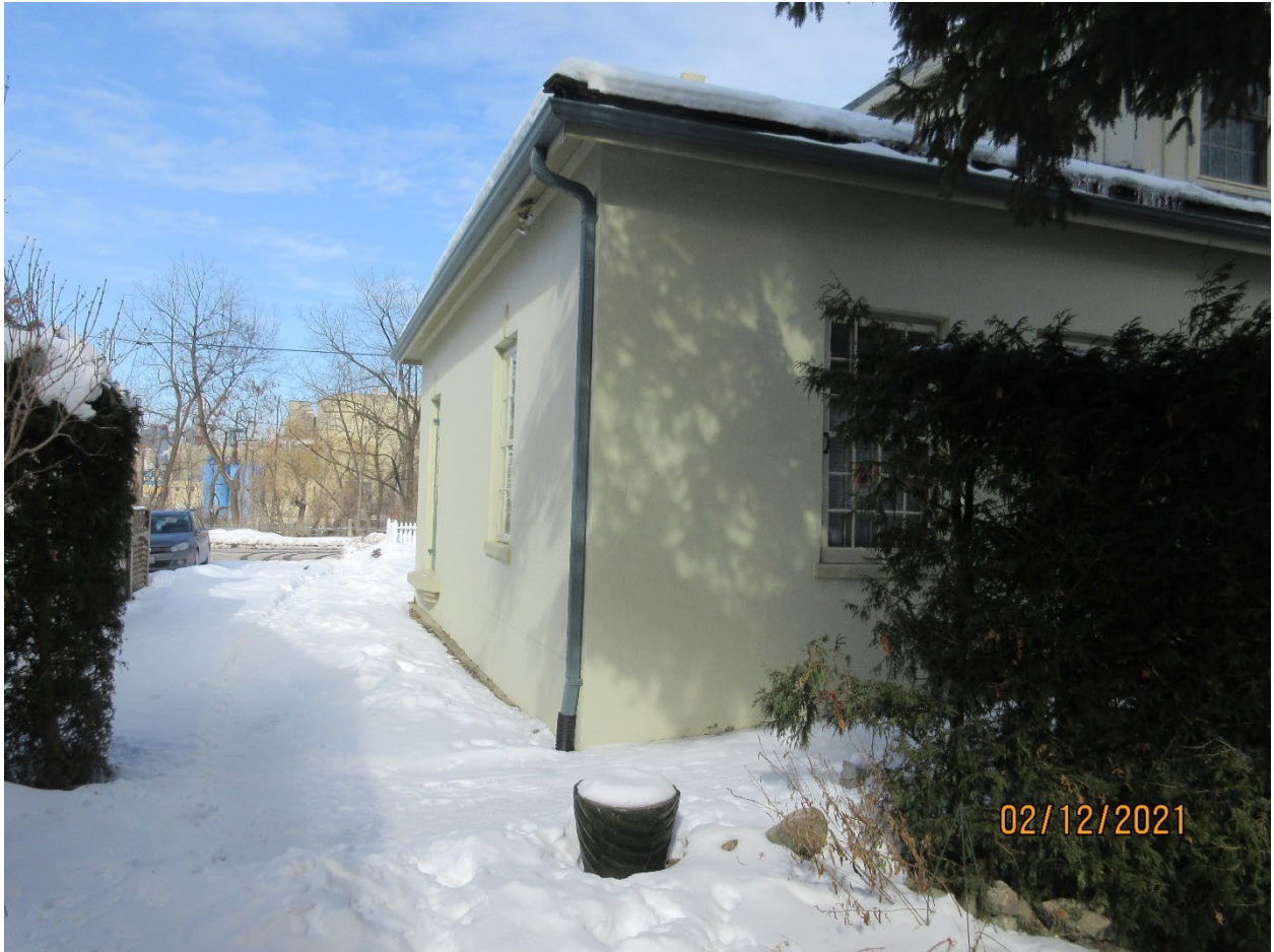
Image 27: View of the west and south facades of Carfrae Cottage, and showing the driveway along the westerly property boundary (2021).
