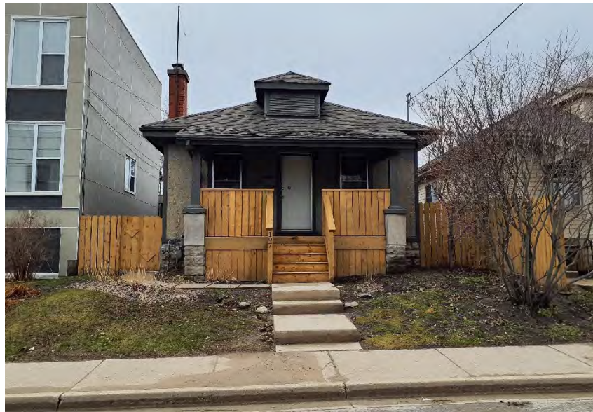
Photo 25: View of front (north) elevation of the building (MHBC, 2023).
