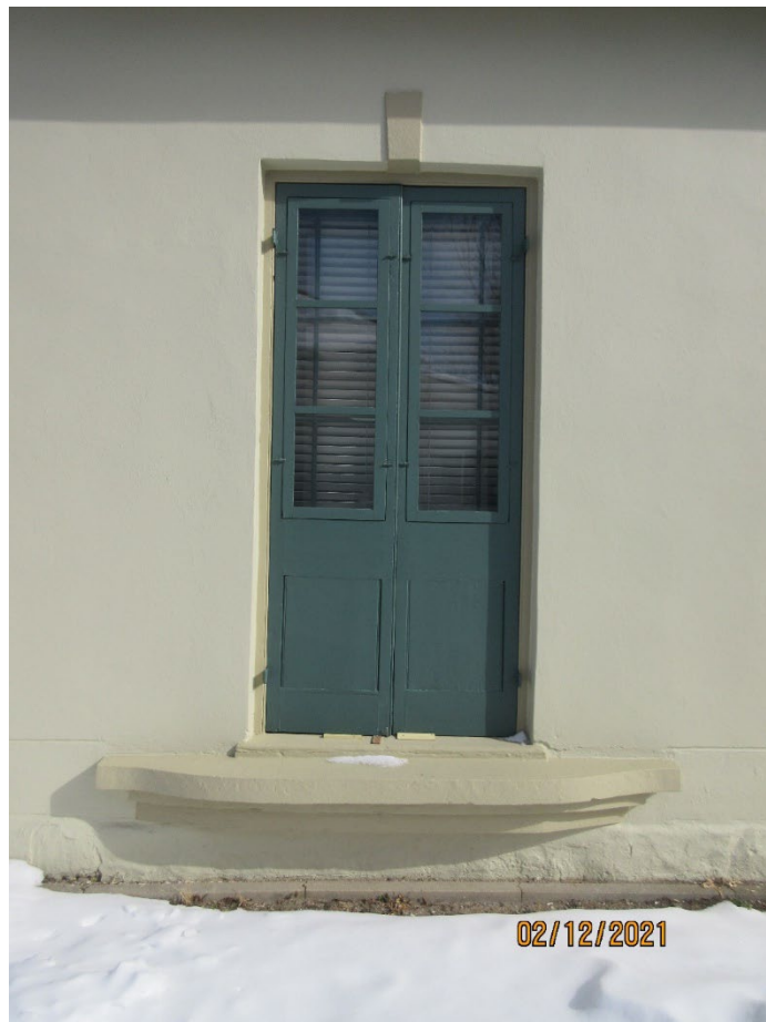
Image 28: Photograph of the painted wood French doors and painted wood storm doors in the opening of the west façade, sill as an indication of the former verandah of Carfrae Cottage (2021).
