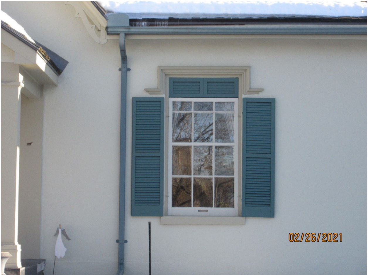
Image 23: Photograph showing the westerly front window, label, and sill of the front (north) façade of Carfrae Cottage (2021).
