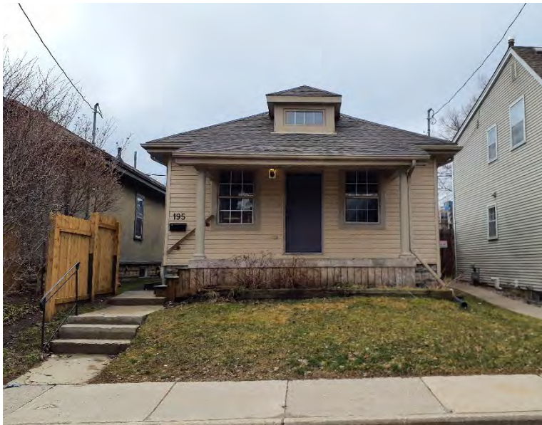
Photo 24: View of front (north) elevation of the building (MHBC, 2023).
