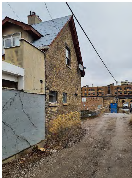
Photos 28-30: (above left) Perspective view of north elevation; (above right) View of south and east elevation (below) View of south and west elevation (MHBC, 2023).
