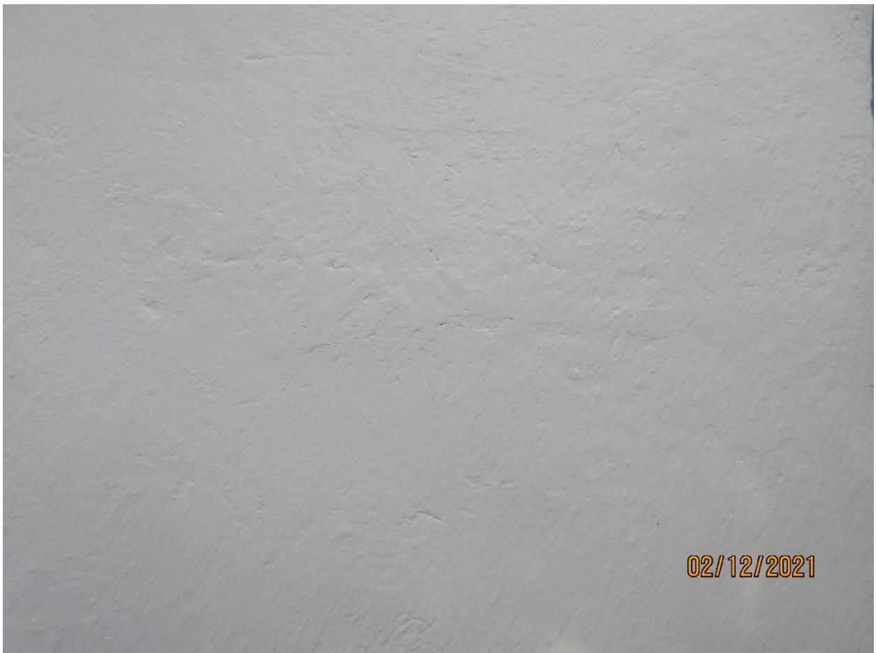
Image 14: Photograph, showing a representative example, of the traditional stucco parging (cementitious smooth textured exterior 'stucco' finish) over the double brick construction of Carfrae Cottage (2021).
