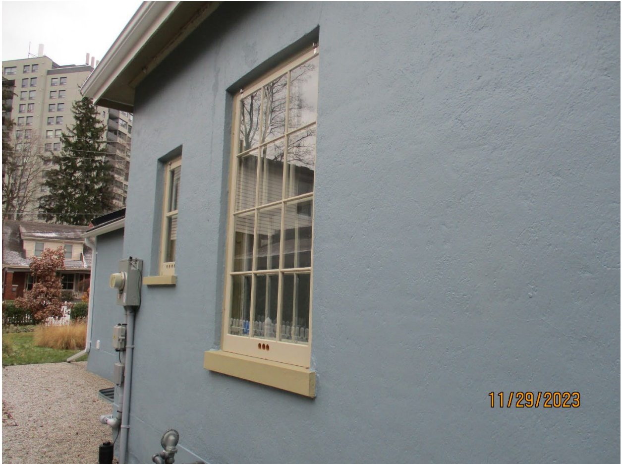
Image 33: Photograph of the painted wood six-over-six shingle hung wood window on west façade (2023).
