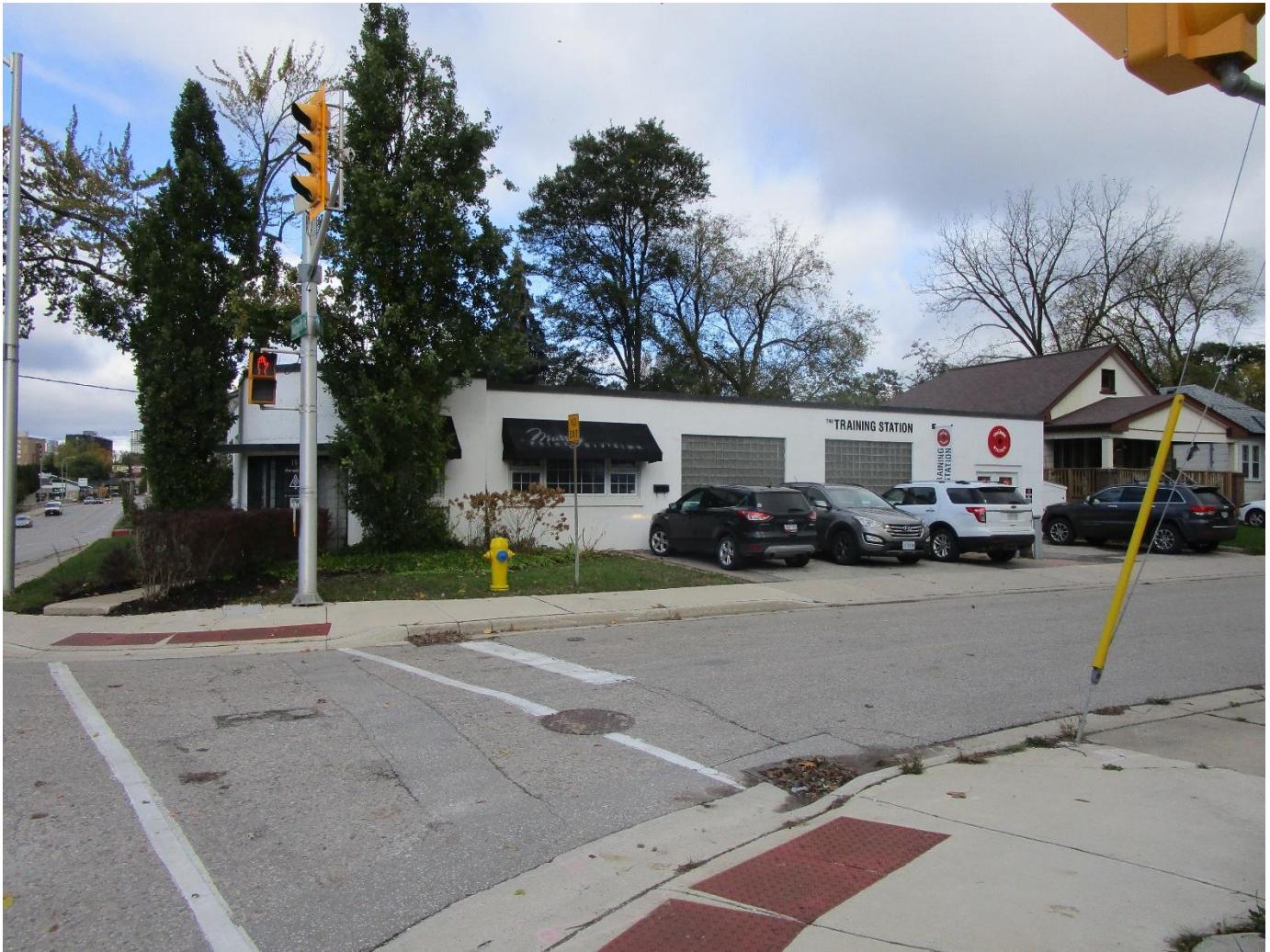
Photograph 1: South elevation of 16 Wellington Road, looking north (AECOM 2021)
