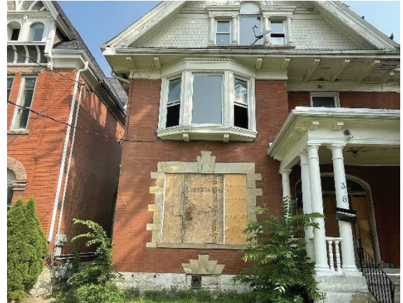
Photo 29: Easternmost bay on south façade
