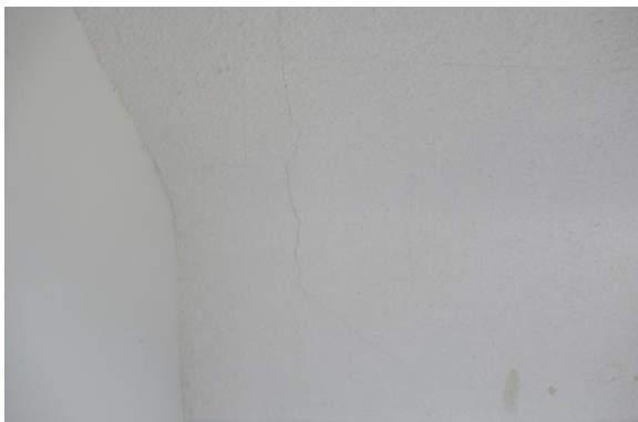
Photo Exhibit No. 21 30 Wellington – large cracks in the ceiling, extending full ceiling length.
