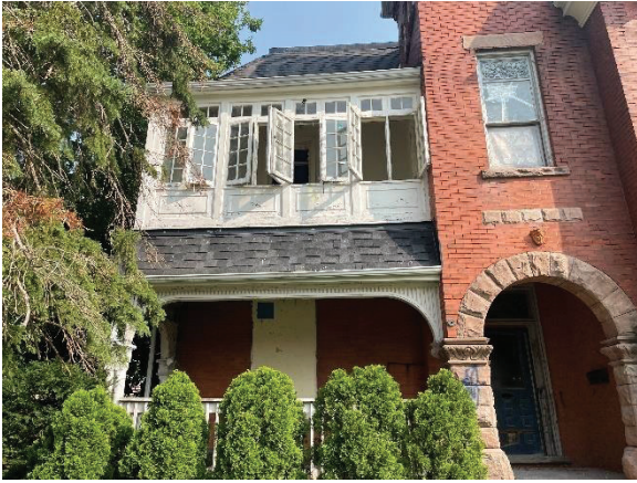
Photo 20: Second storey enclosed balcony with casement windows in the western bay, looking north
