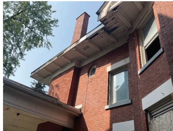
Photo 39: Oval and rectangular windows, east façade
