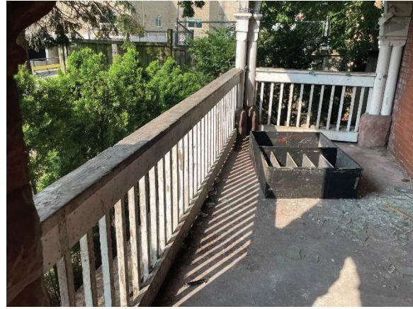
Photo 21: Porch support columns and baluster, looking west
