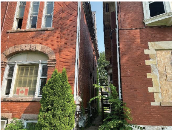
Photo 22: Eastern façade, looking north
