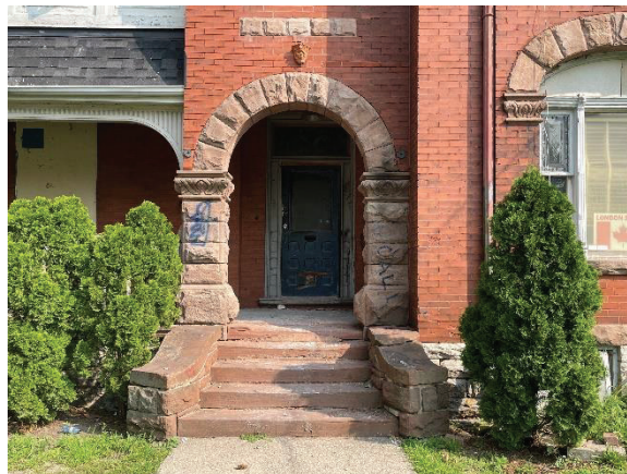
Photo 15: Stairs and arch leading to the residence's main entrance, looking north
