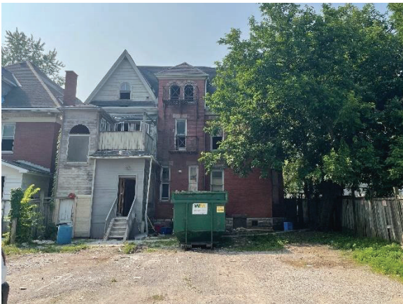
Photo 26: North façade, looking south
