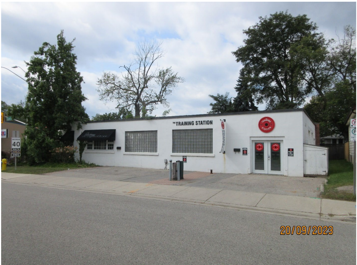
Image 2: Photograph of the south elevation of the building on the subject property at 16 Wellington Road (taken September 20, 2023).
