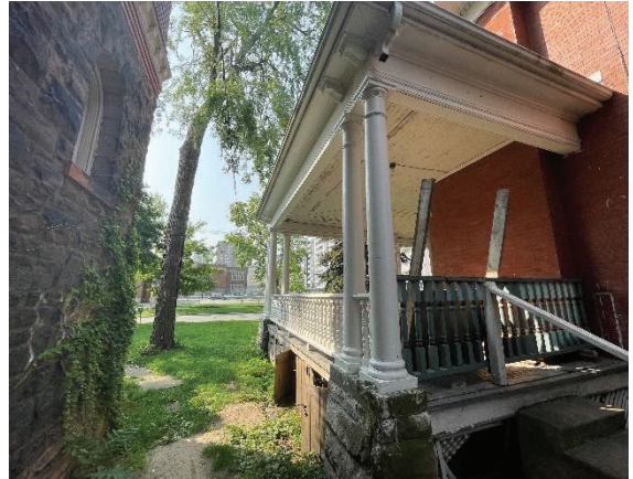
Photo 41: East façade wrap-around porch
