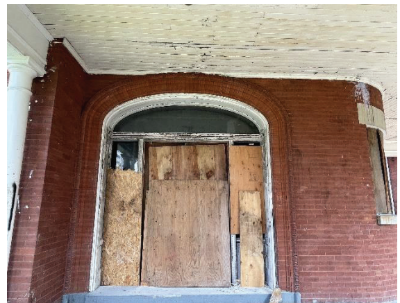
Photo 31: Front entrance door
