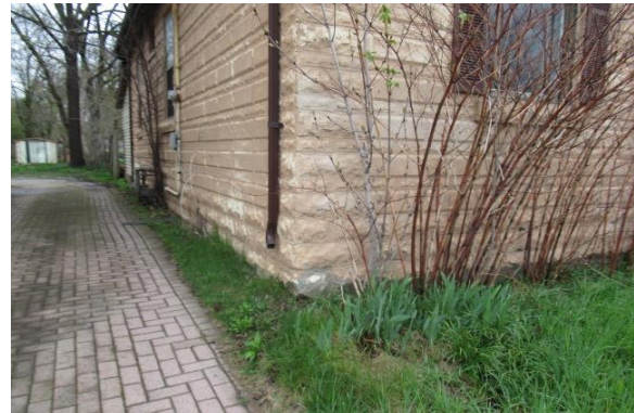
Photo Exhibit No. 23 30 Wellington – exterior façade bricks extend below grade but support the bricks above.
