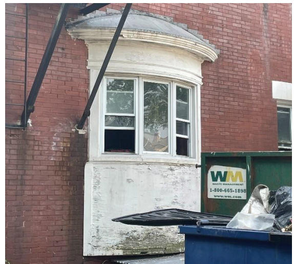
Photo 43: Curved bay window, north façade
