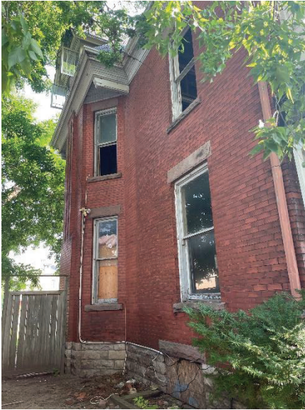
Photo 24: Western façade, looking northeast
