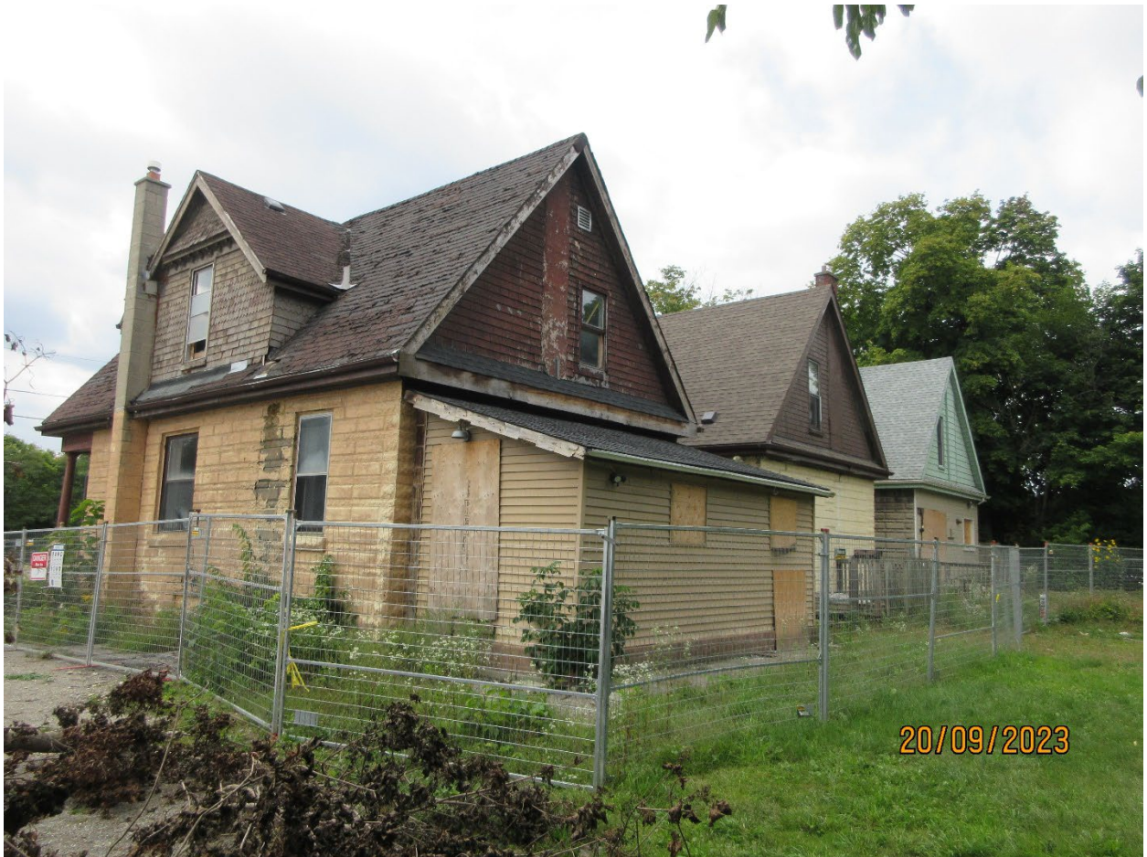
Image 8: Photograph showing the buildings on the subject properties at 26-28-30 Wellington Road (taken September 20, 2023).
