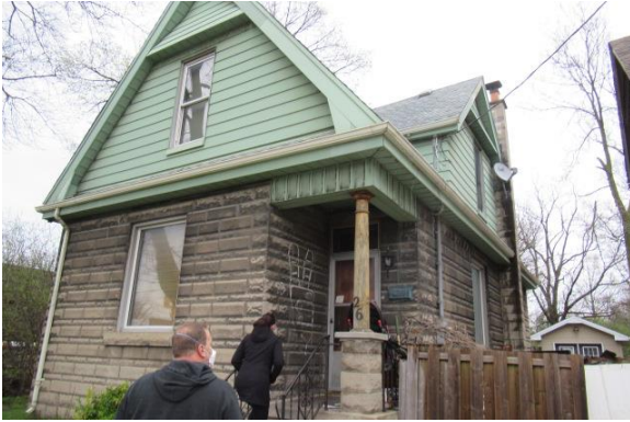
Photo Exhibit No. 1 26 Wellington – front elevation.
