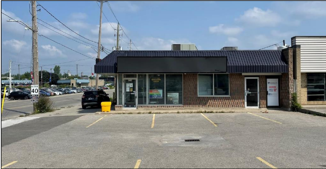
Figure 2 - Streetview of 1544 Dundas Street (view looking North)
