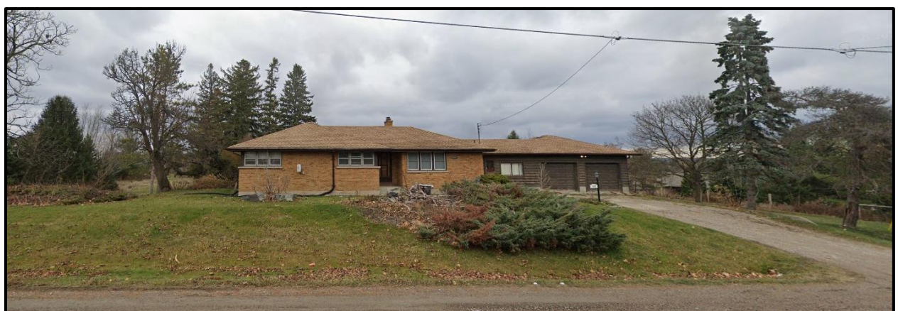
Figure 2. Streetview of 1982 Commissioners Road East (view from Commissioners Road East).
