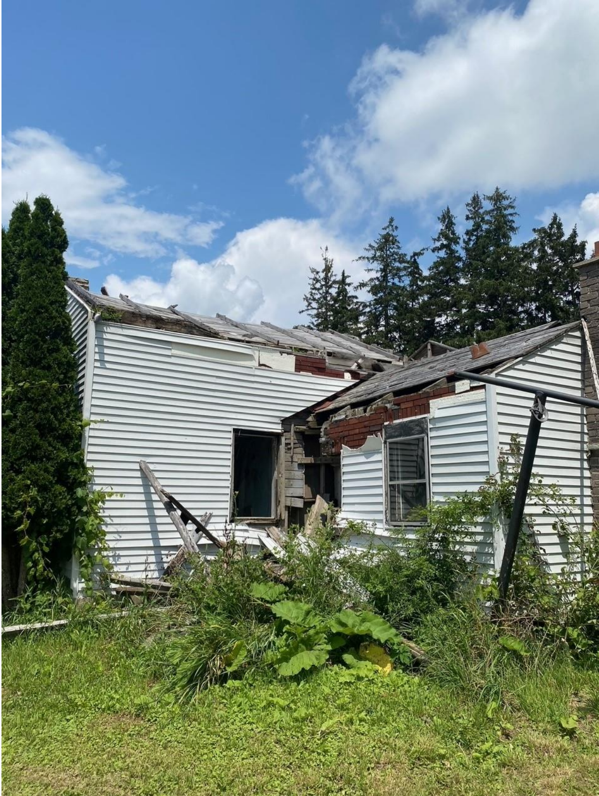
1803 Bradley Ave – Rear Exterior
