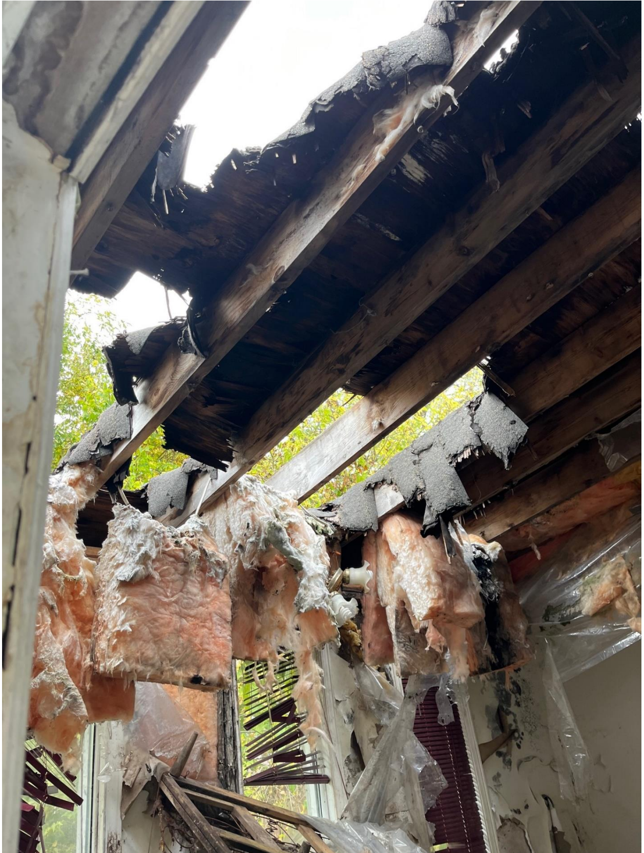
19 Redan St – Interior & Roof Example
