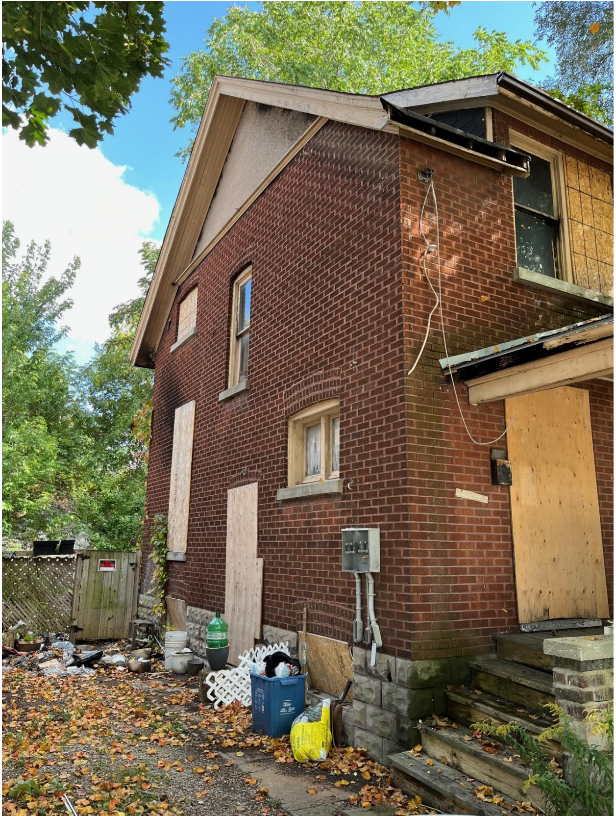
712 Adelaide St N – North Side
