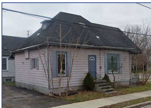
3.(top left) East elevation. 4, (top right) North-East elevation.
