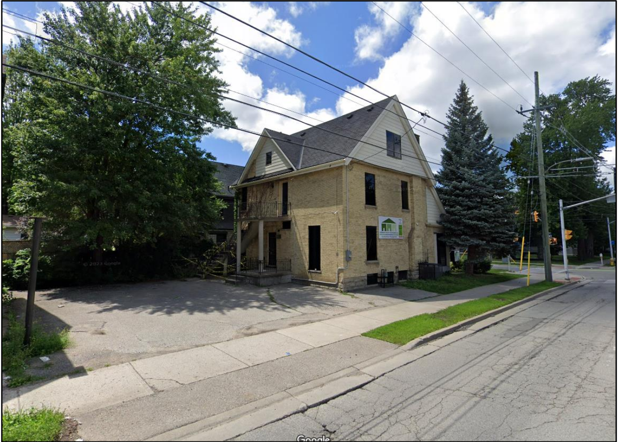
Figure 2 - Streetview of 607 Queens Avenue from Adelaide Street (view looking west)
