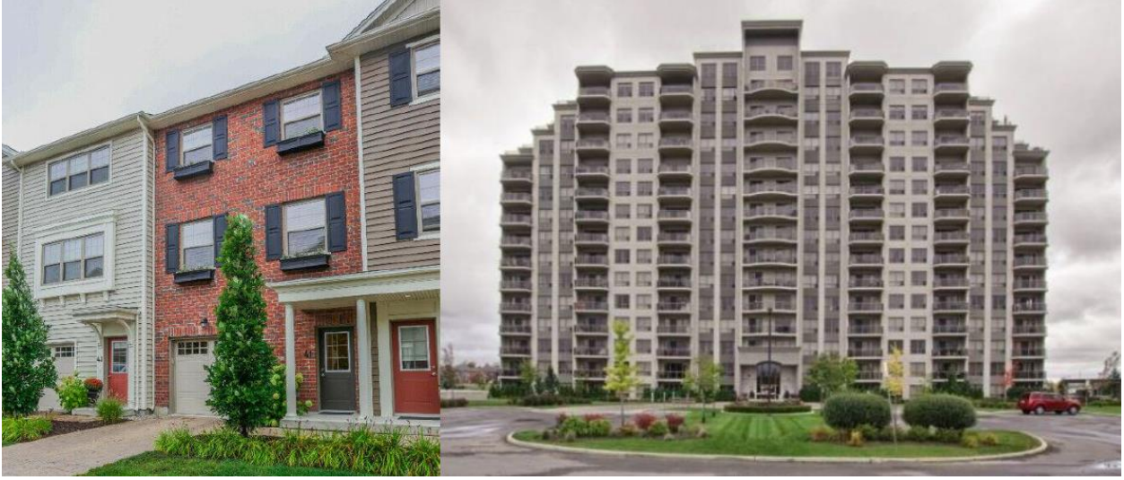
Figure 2: Apartment building and townhomes to the south
