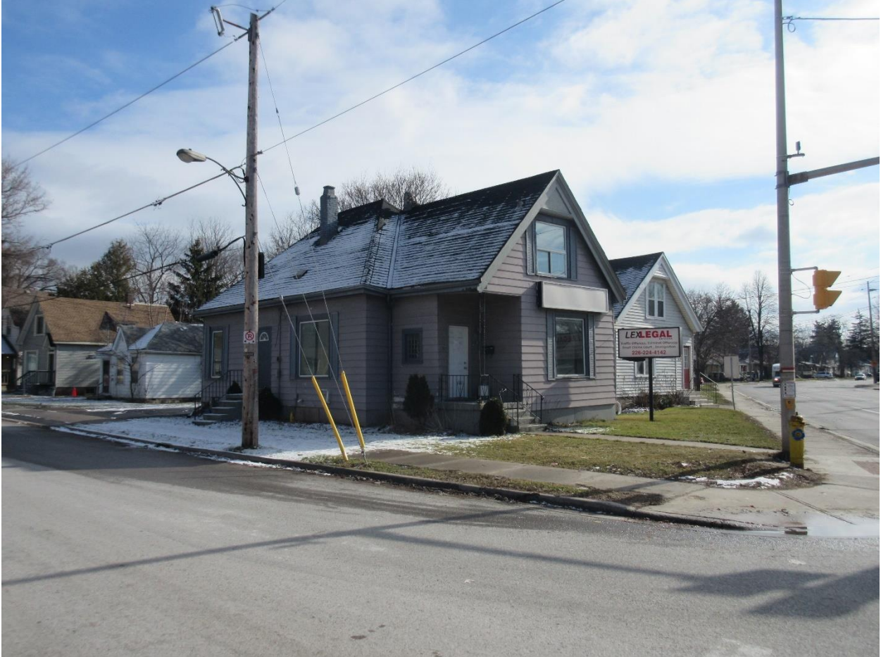
Image 1: Northwest corner of the Contributing Resource at 187 Wharncliffe Road North (taken February 5, 2016).
