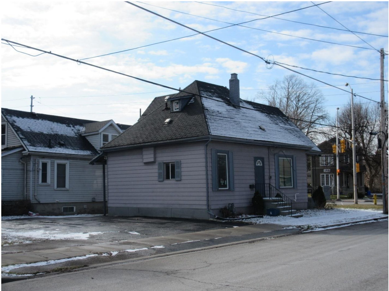
Image 3: Northeast corner of the Contributing Resource at 187 Wharncliffe Road North (taken February 5, 2016).
