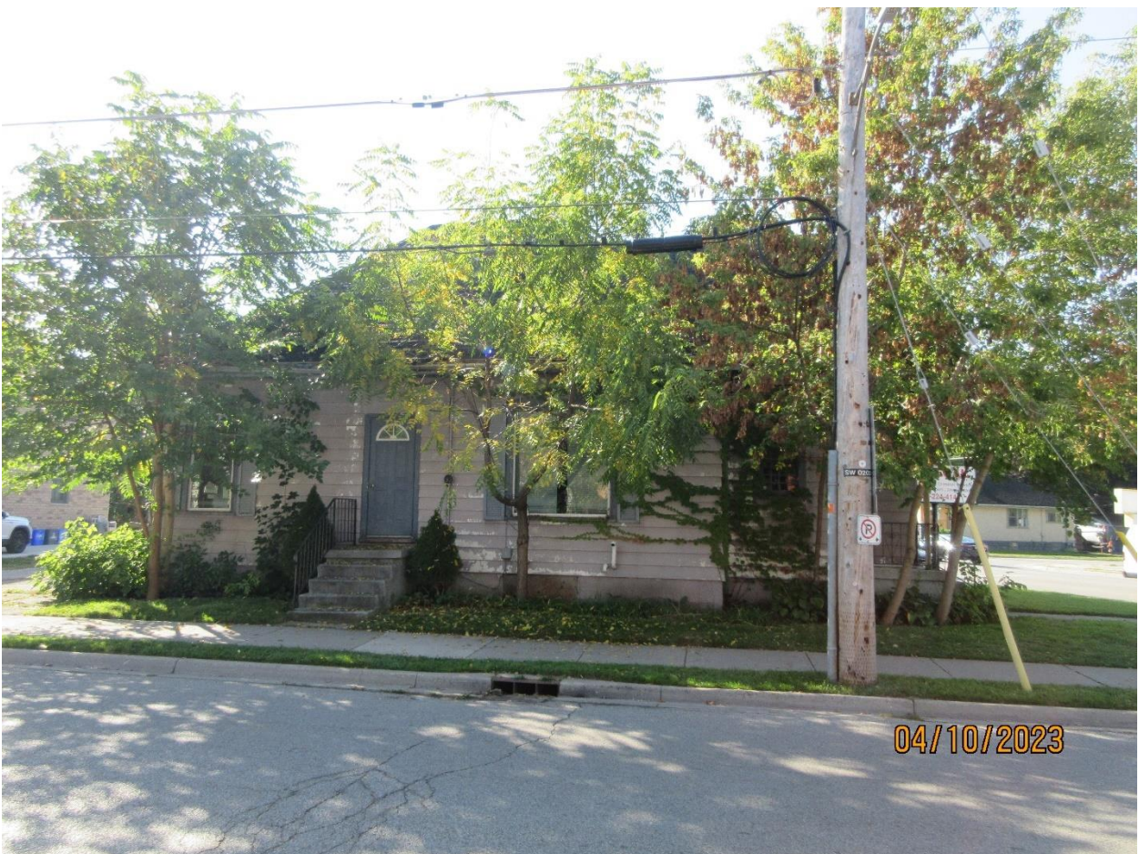
Image 7: North elevation of the Contributing Resource at 187 Wharncliffe Road North (taken October 4, 2023).
