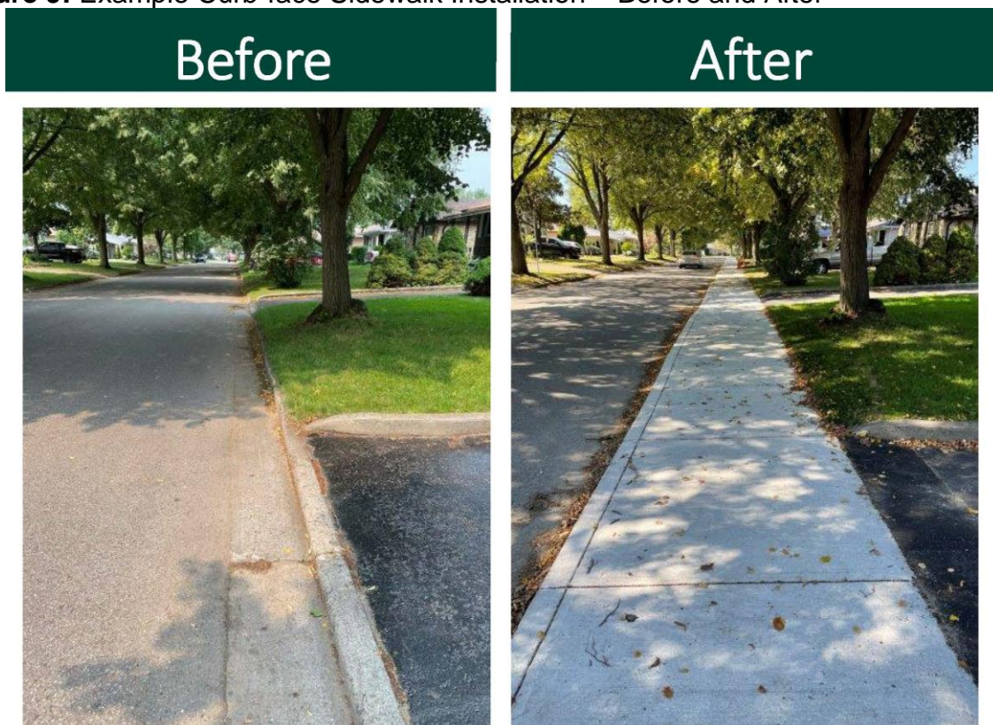
Figure 9: Example Curb-face Sidewalk Installation – Before and After
