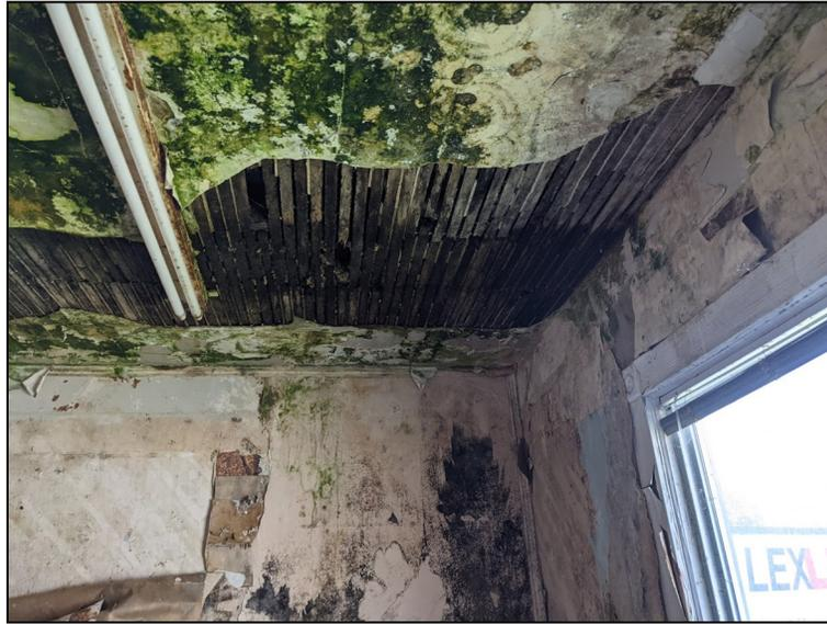
**Photograph 3 – Damaged Upper Floor Framing**
