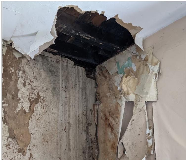
Photograph 1 - Interior finish damage
