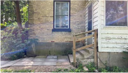
79. 7056 Pack Rd East Facade Mud Room Addition & Concrete Foundation Work.HEIC
