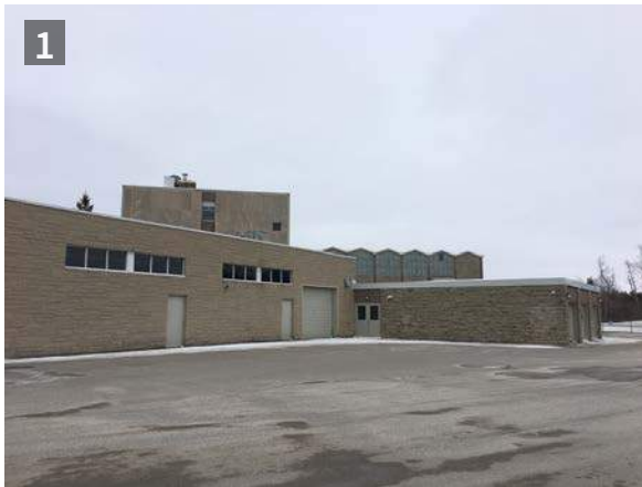
Looking northeast towards 1987 technology wing addition (ERA, 2018).
