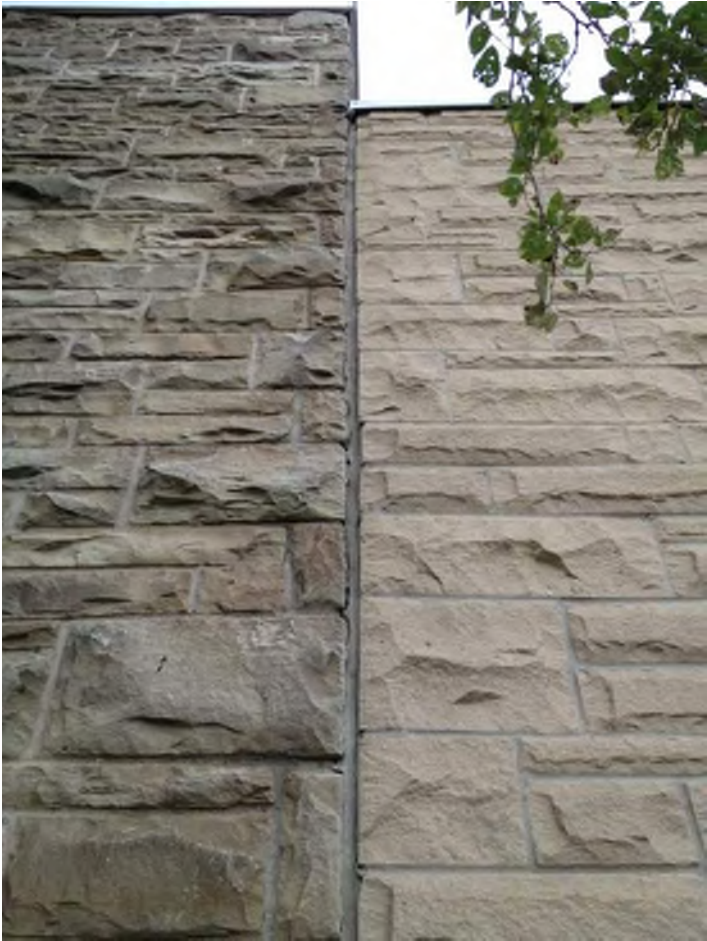
Caulked expansion joint at tech wing addition
