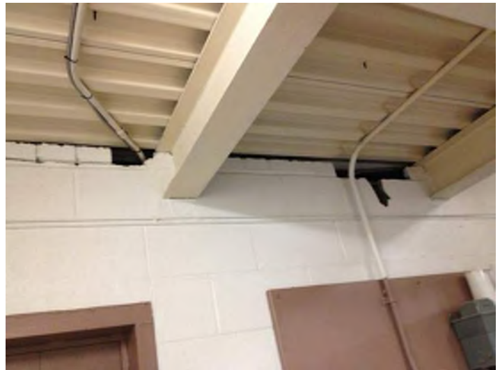
Fire separation at elevator machine room
