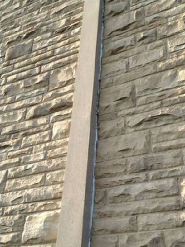
Caulked joint at Gymnasium wall - South Elevation
