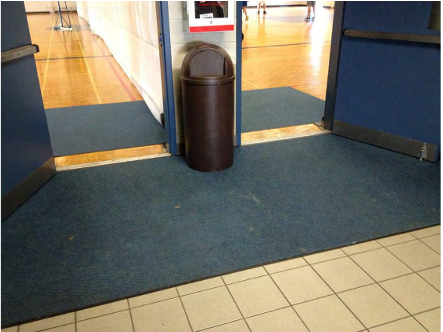
Gymnasium interior entrance - replacement of wood floor in Gymnasium with new will require alterations to door frames along with tapering flooring leading into Gymnasium.
