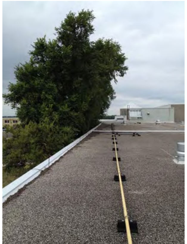
Overhanging trees at Roof H
