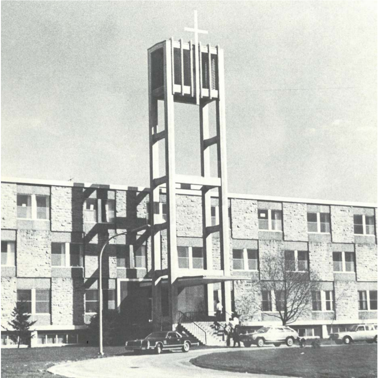
Original main entry and bell tower (demolished) (London District Catholic School Board, year unknown).
