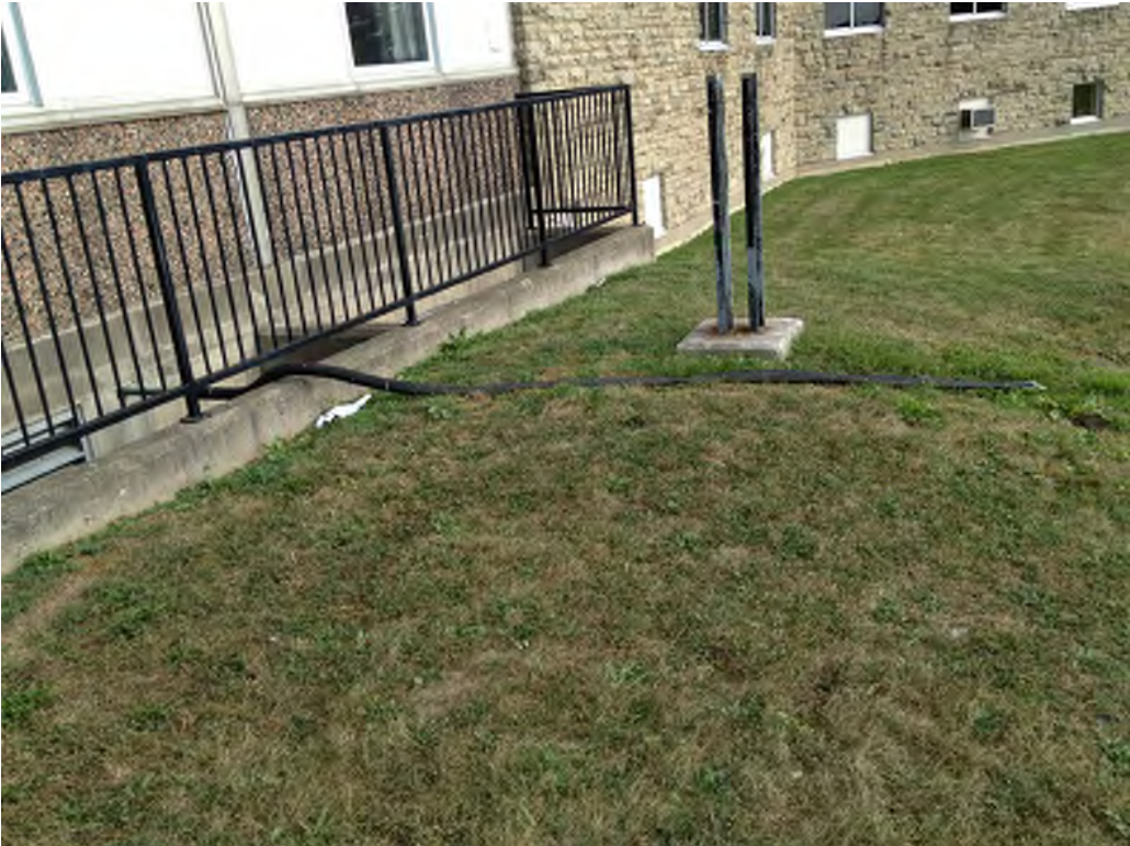
Drain pipe at west elevation
