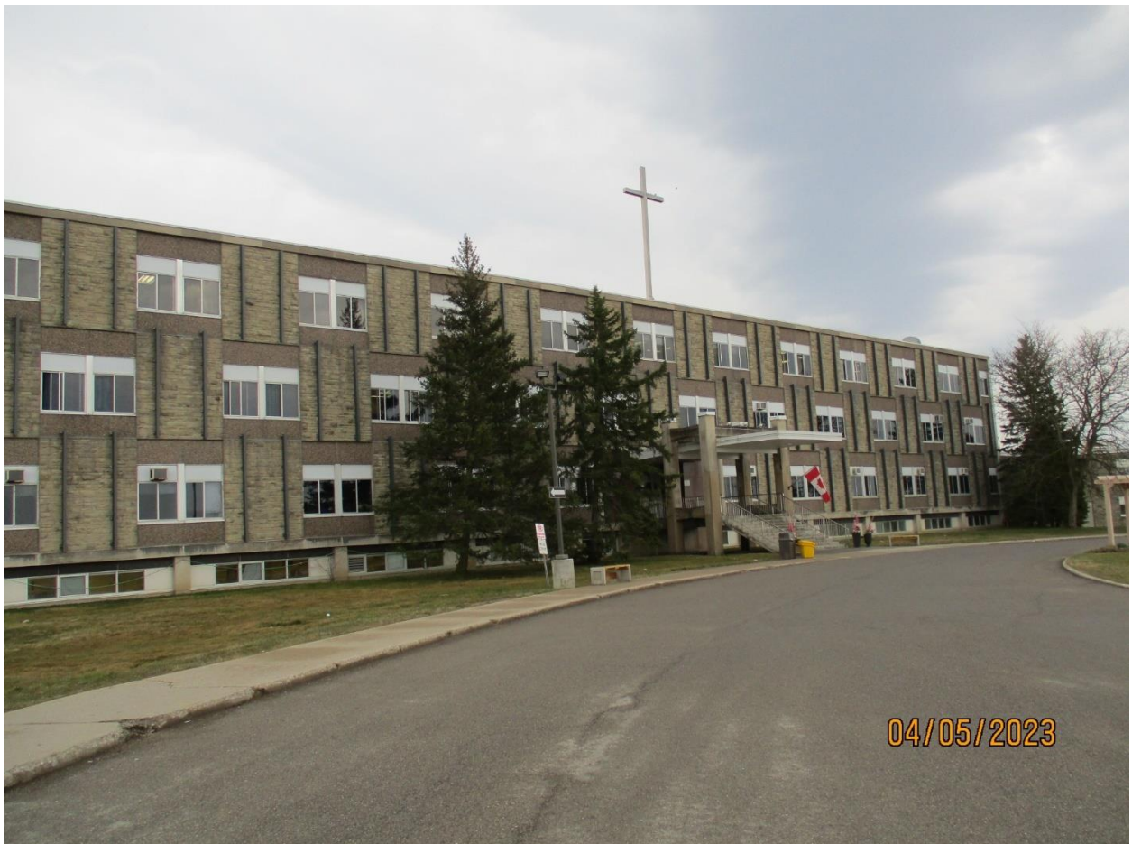
Image 2: Photograph showing the west (front) façade of the Regina Mundi Catholic College at 5200 Wellington Road South.
