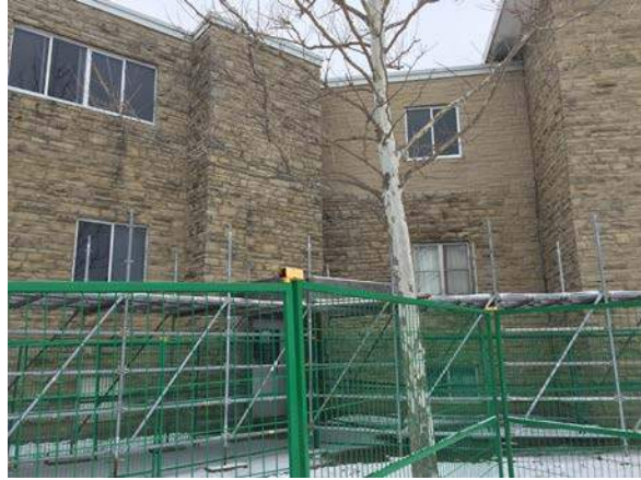
Scaffolding installed over door at east elevation, beside the “gymnasium” (ERA, 2018).
