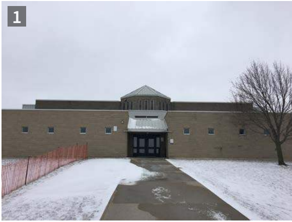
1987 north gymnasium addition (ERA, 2018).
