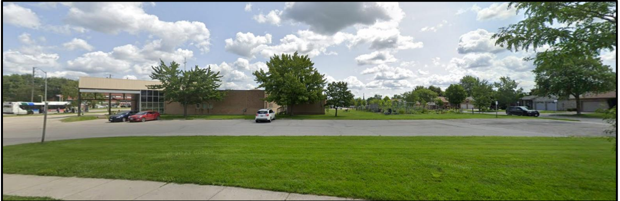
Figure 3. Streetview of 1901 Jalna Boulevard (view from Jalna Boulevard looking west)
