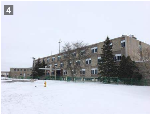
Looking east towards the school (ERA, 2018).
