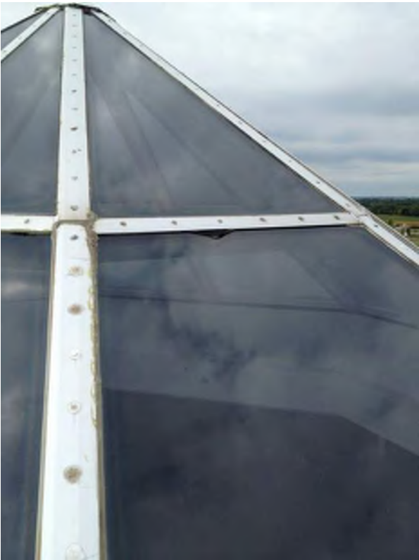
Library skylight exterior
