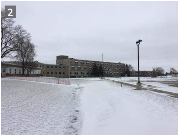
Looking south towards the school (ERA, 2018).
