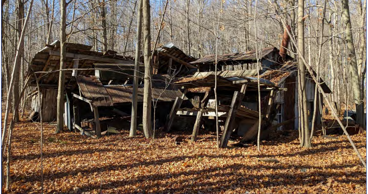
Photo 45: View of the southeast elevation
