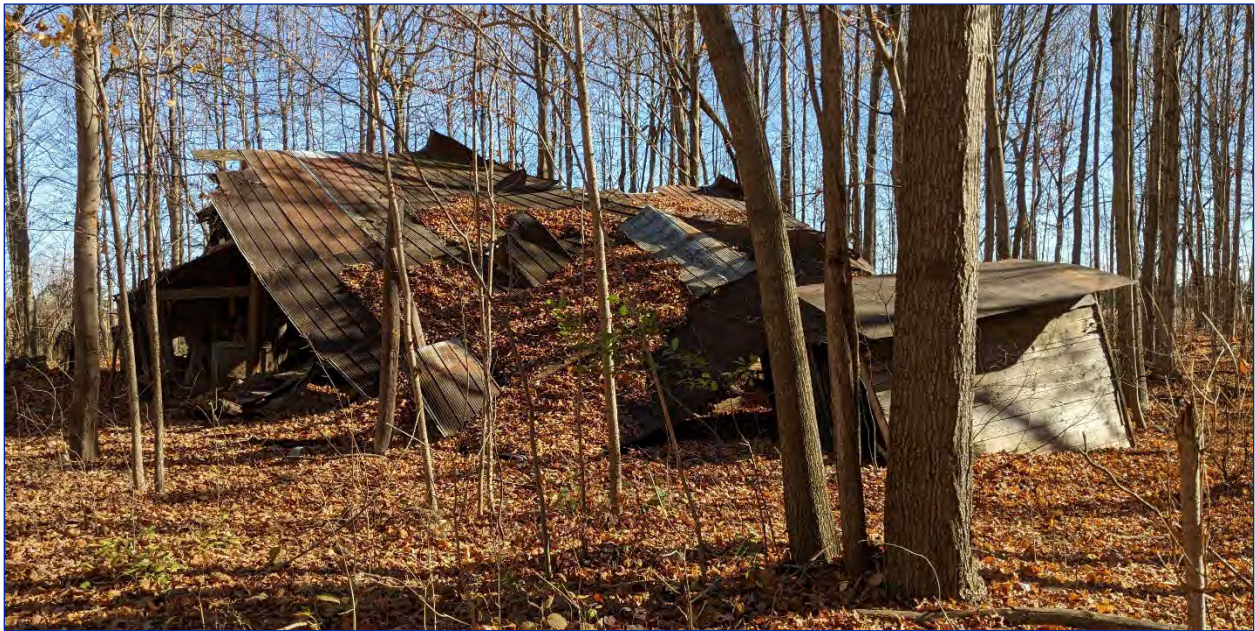
Photo 42: View of the west elevation
