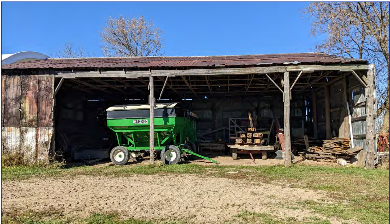
Photo 25: View of the south elevation
