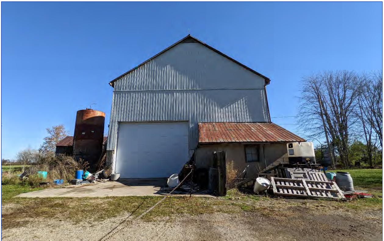
Photo 17: View of the west elevation
