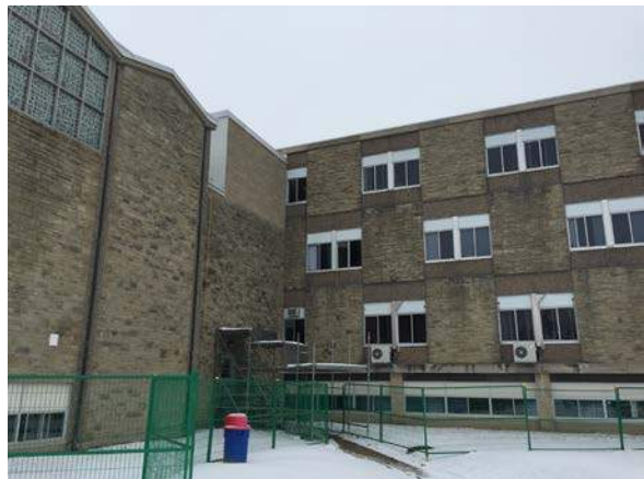
Scaffolding installed over door at north chapel elevation (ERA, 2018).
