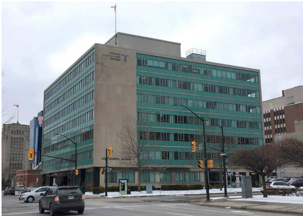
Crown Trust Building (1957), 200 Queens Avenue, London. Robert Buist for Watt & Tillmann (ERA, 2018).
