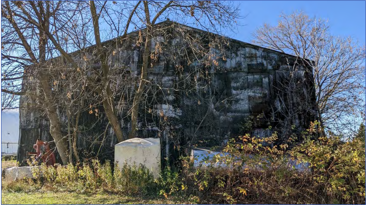
Photo 24: View of the east elevation
