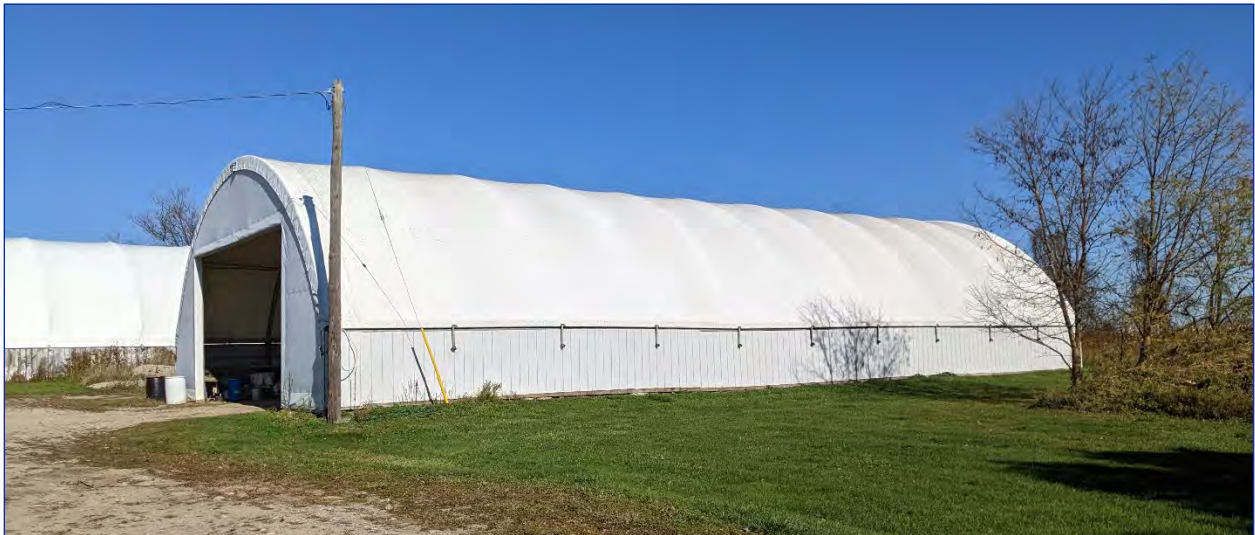
Photo 26: View of the south and west elevations
