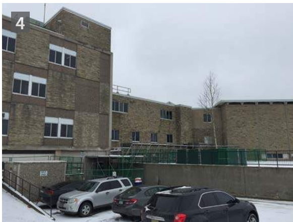
Looking north towards rear elevation of school and "gym-torium" wing (ERA, 2018).
