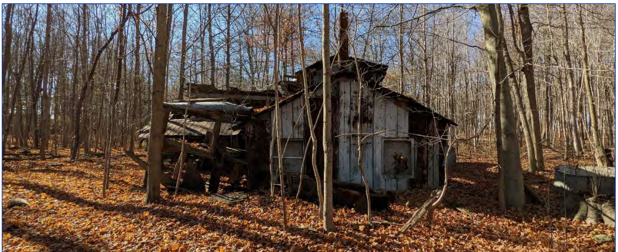
Photo 44: View of the east elevation
