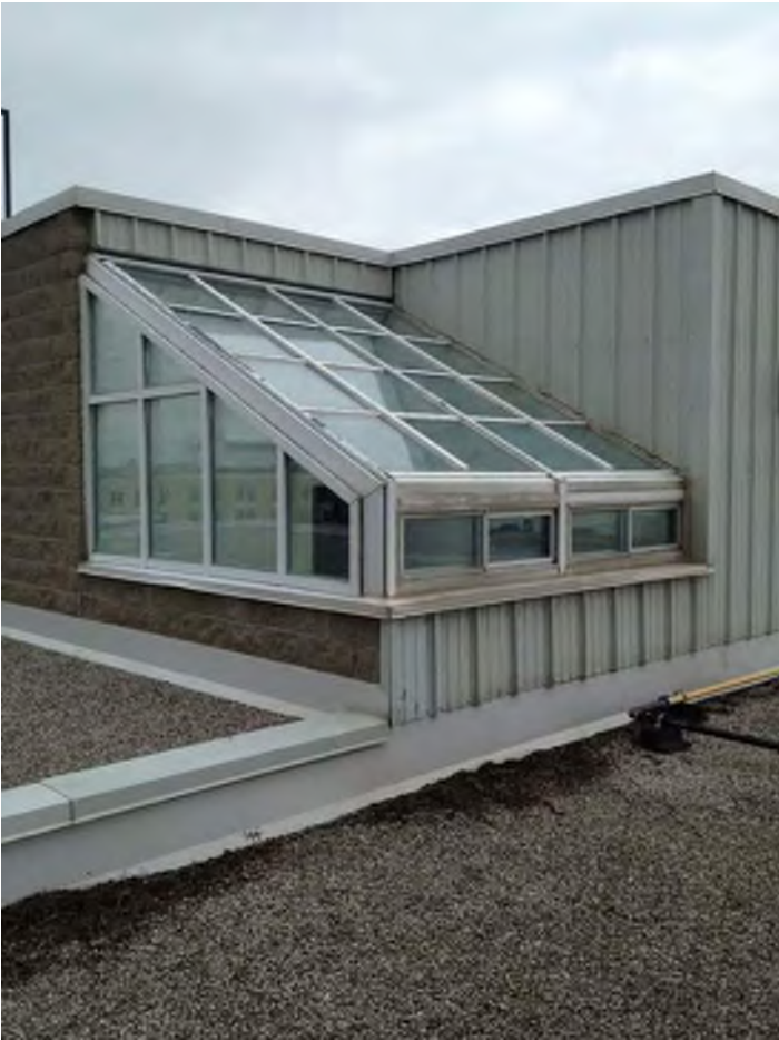
Overall exterior greenhouse structure
