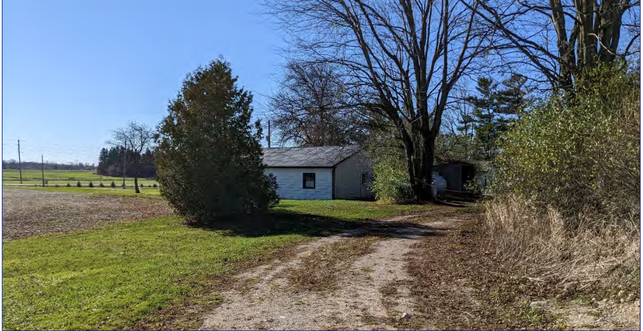
Photo 35: View of the northeast elevation
