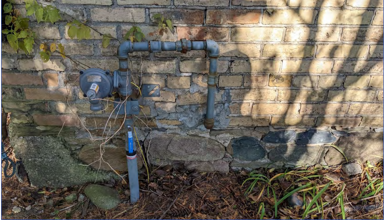
Photo 14: Detailed view of the field stone foundation
