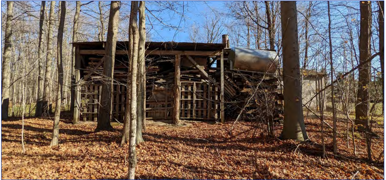
Photo 39: View of the west elevation
