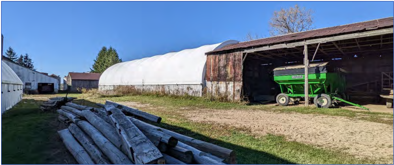
Photo 28: View of the south elevations
