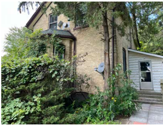
86. 7056 Pack Rd Front Facade Bay Window & Mud Room Addition.HEIC
