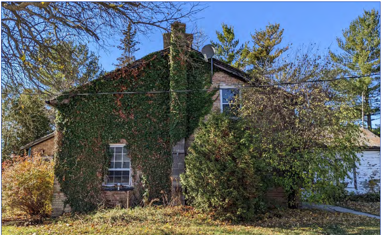
Photo 13: View of the east elevation
