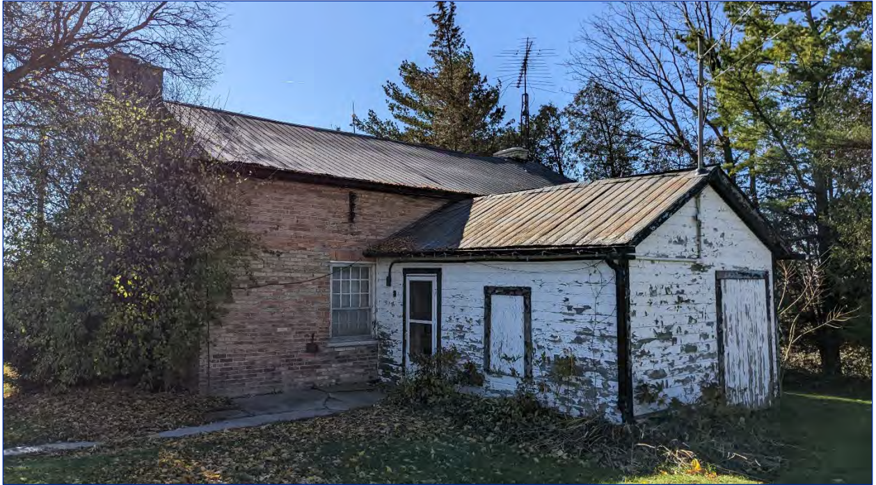
Photo 12: View southwest of the back wall and rear wing of the house
