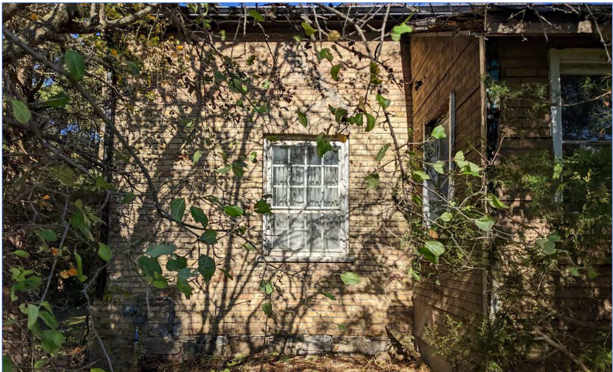
Photo 9: View north of the western half of the south elevation
