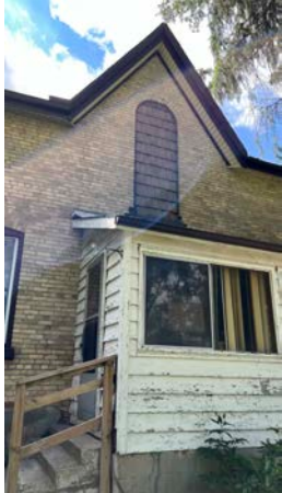
80. 7056 Pack Rd East Facade Boarded Over Window Opening.HEIC
