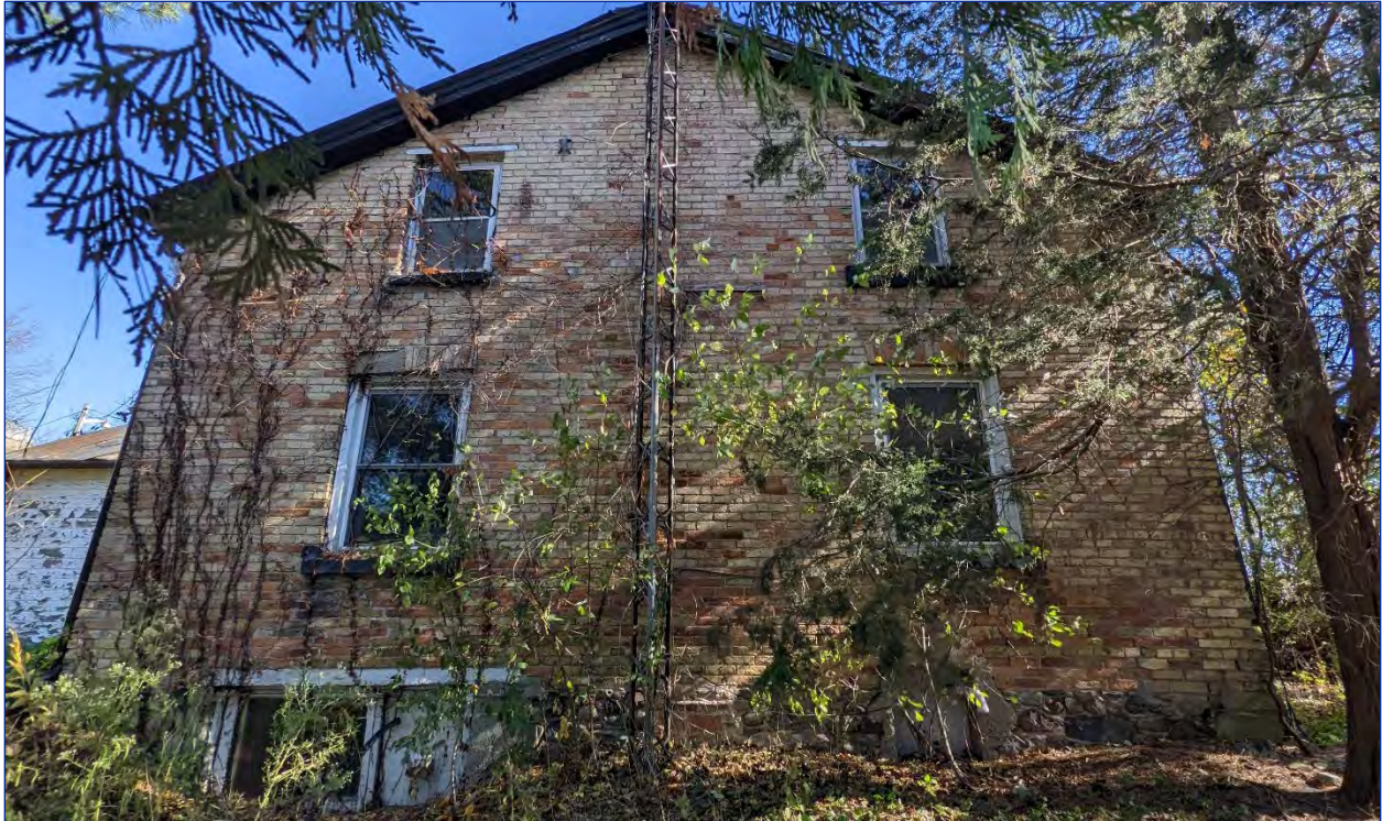
Photo 10: View east of the west elevation
