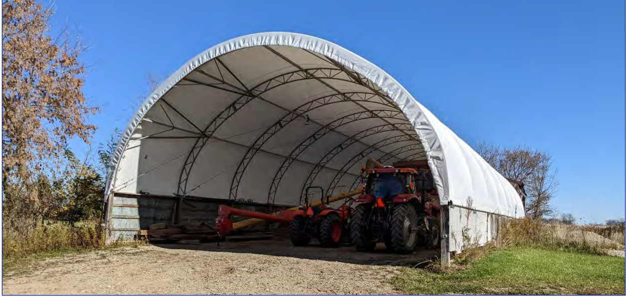
Photo 29: View of the east elevation and the interior
