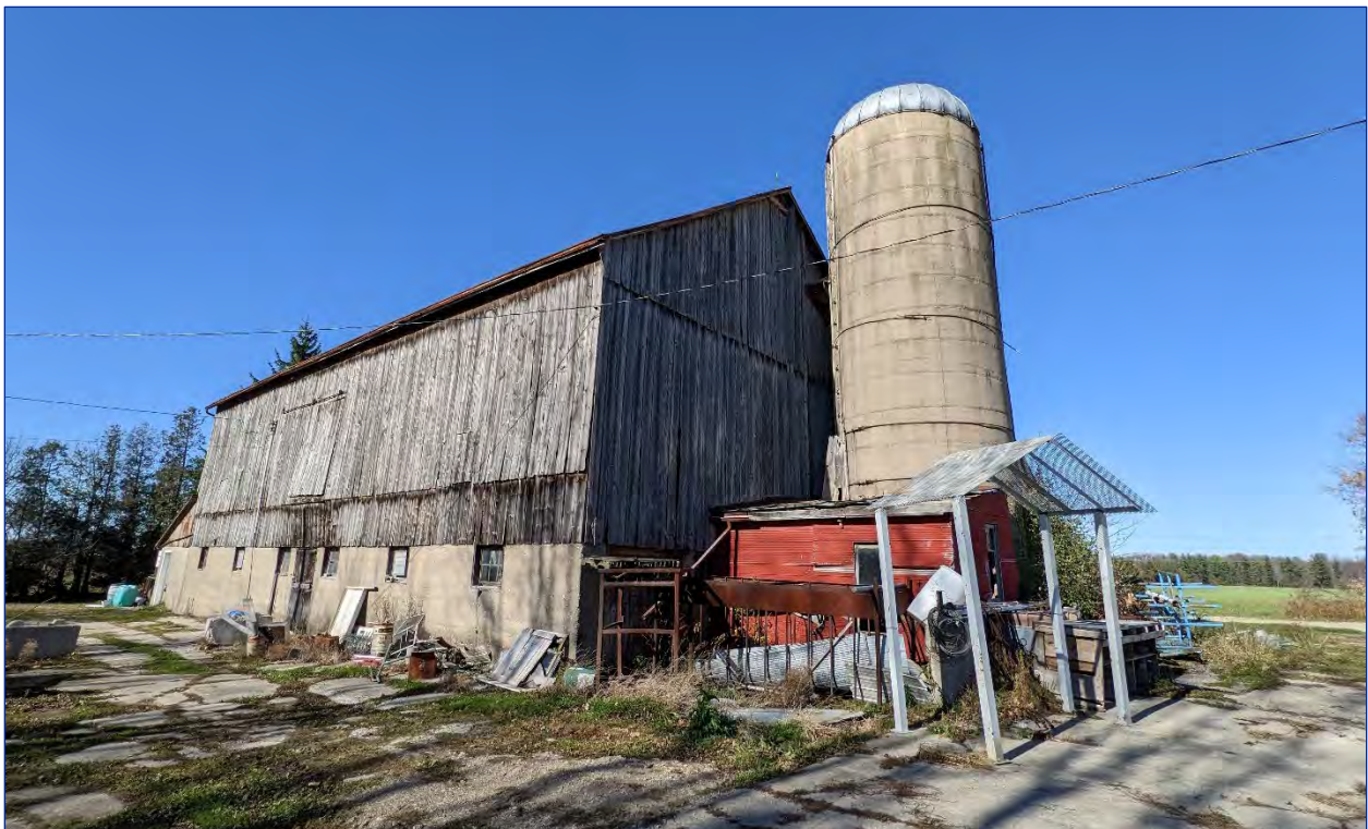
Photo 19: View of the southeast elevation
