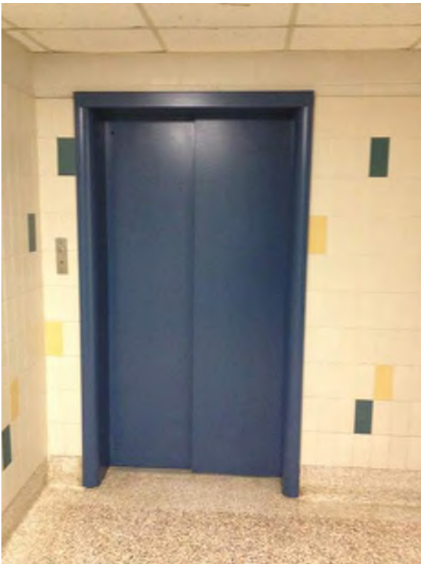
Elevator at Lower Floor
