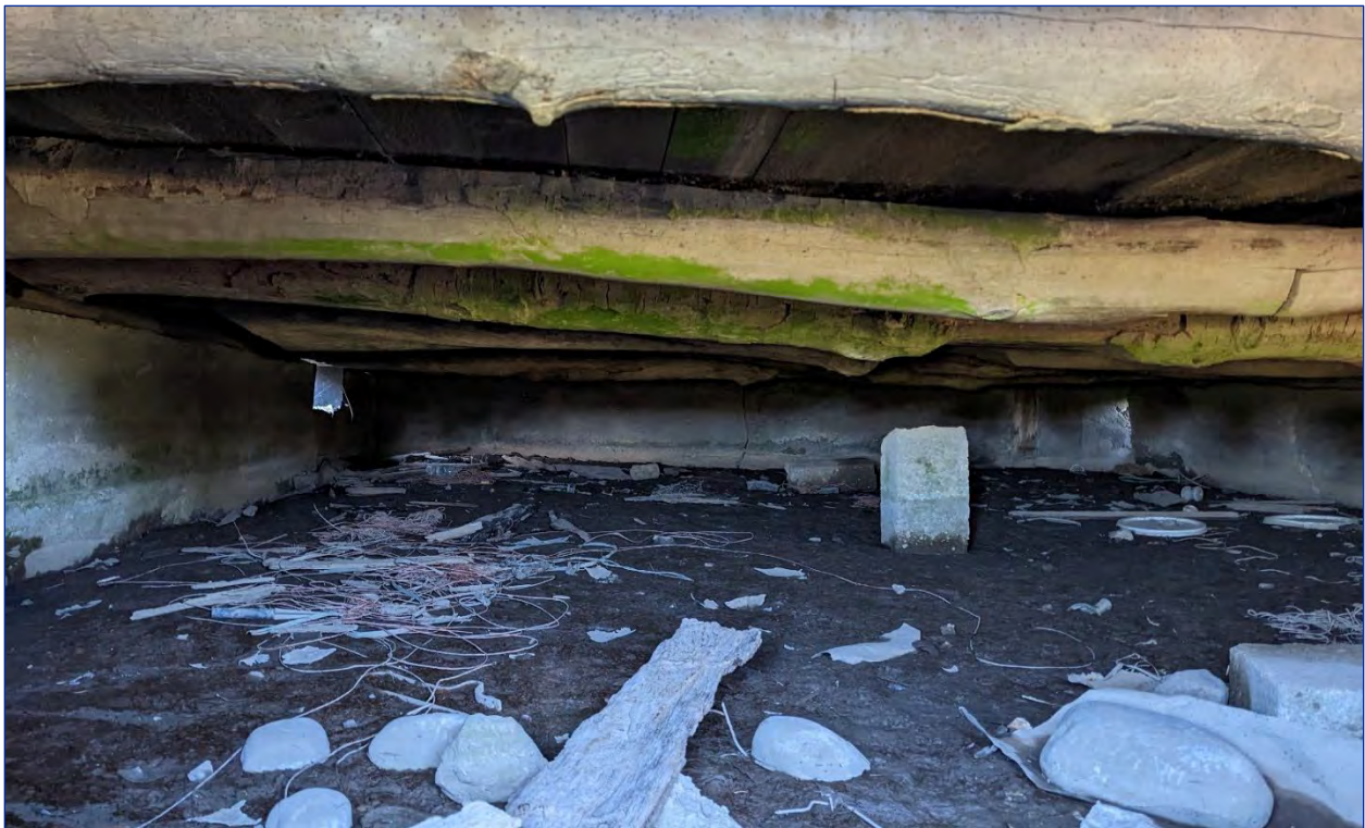
Photo 33: Detail view of the interior of the foundation
