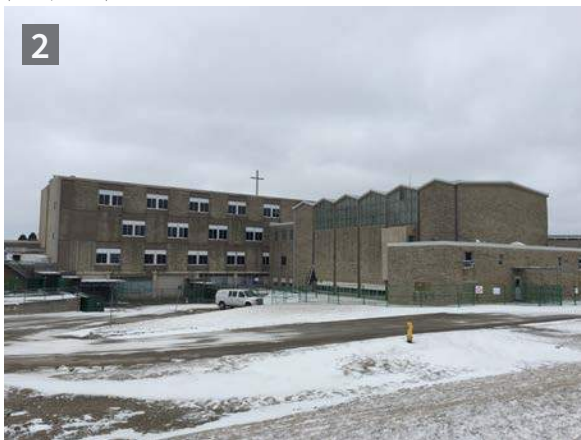
Looking north towards rear elevation of school and chapel (ERA, 2018).
