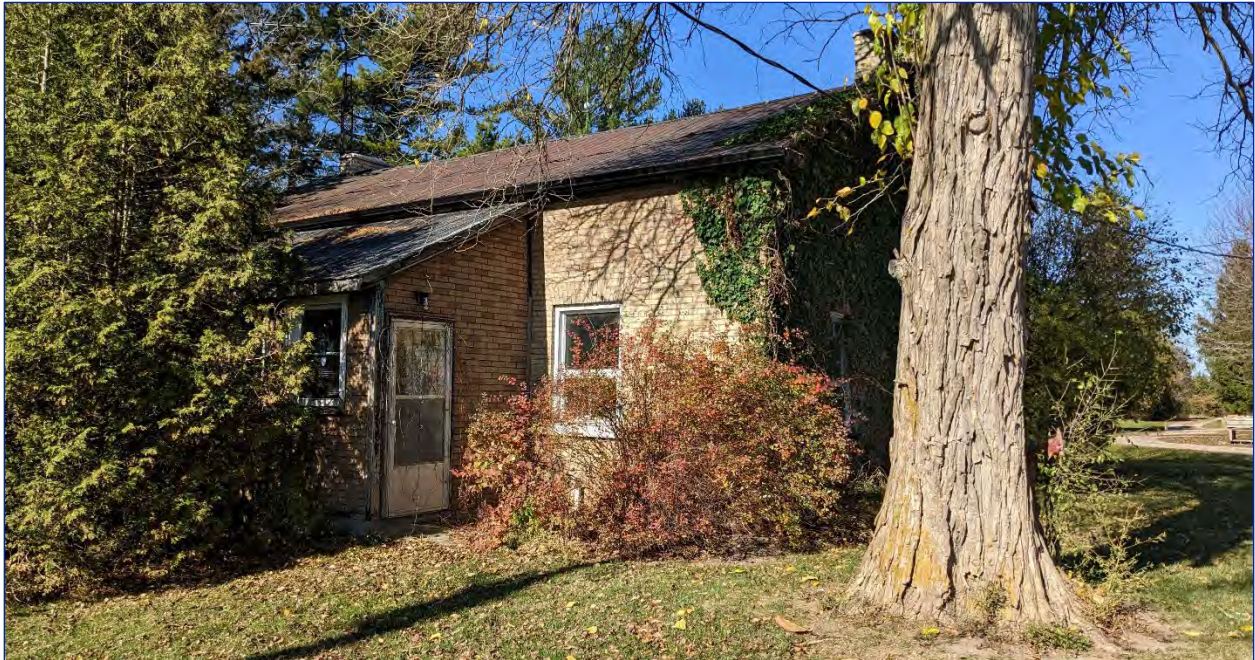
Photo 8: View northwest of southeast elevation of residence
