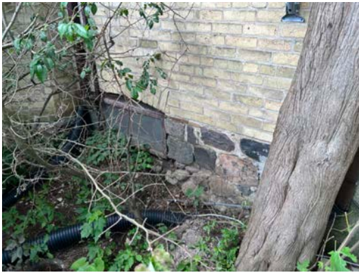
93. 7056 Pack Rd Stone Foundation.HEIC
