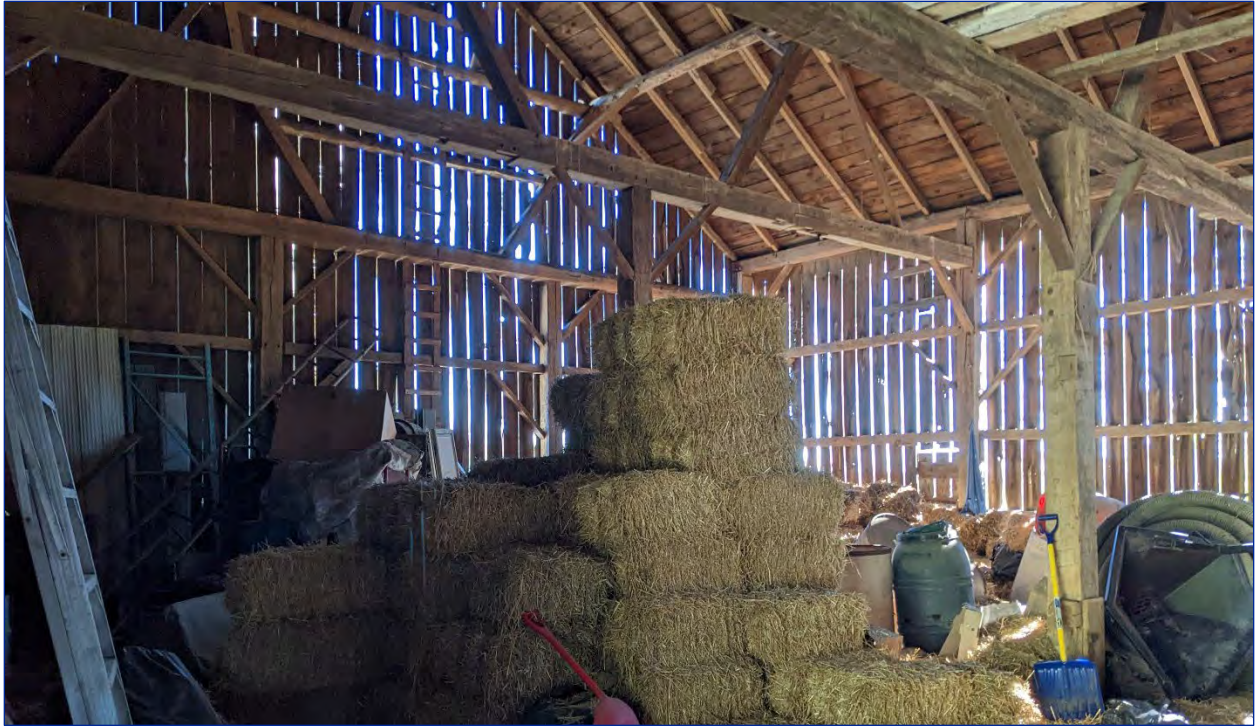
Photo 20: View east of interior
