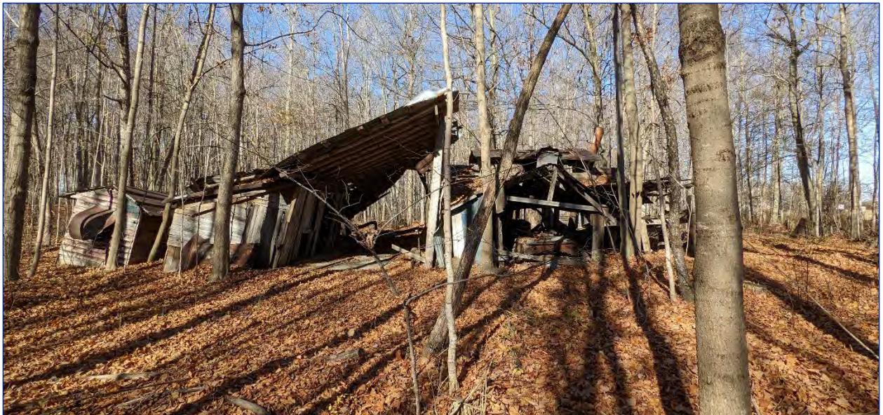
Photo 46: View of the south elevation
