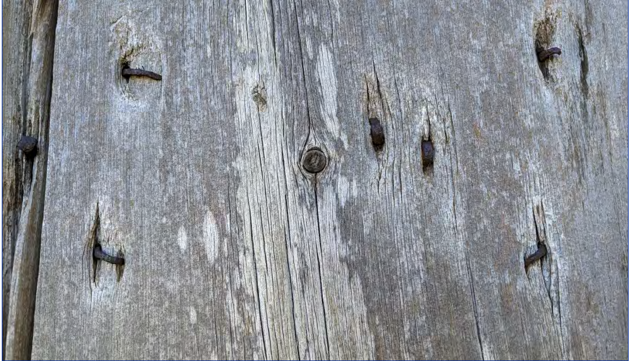
Photo 34: Detailed view of fasteners
