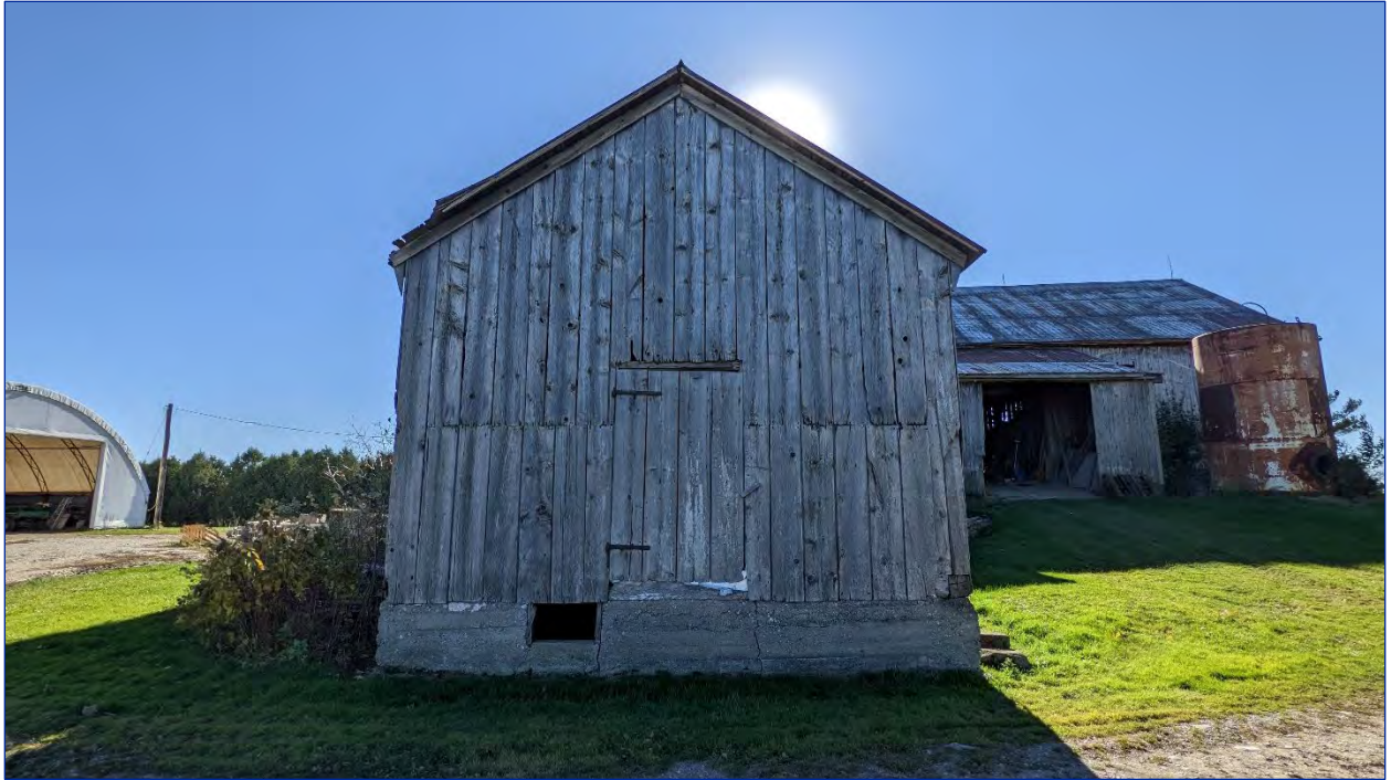
Photo 30: View of the north elevation
