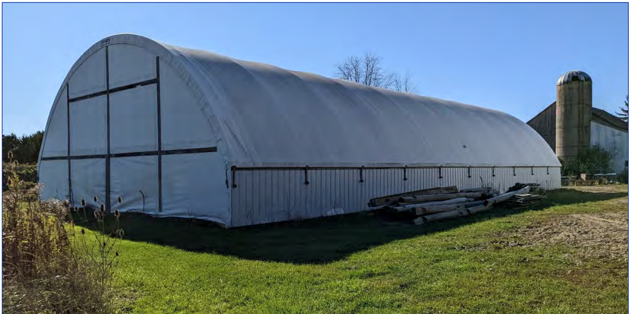
Photo 27: View of the north and east elevations
