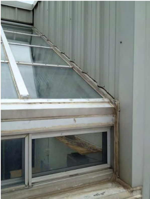
Greenhouse interface with adjacent wall.
