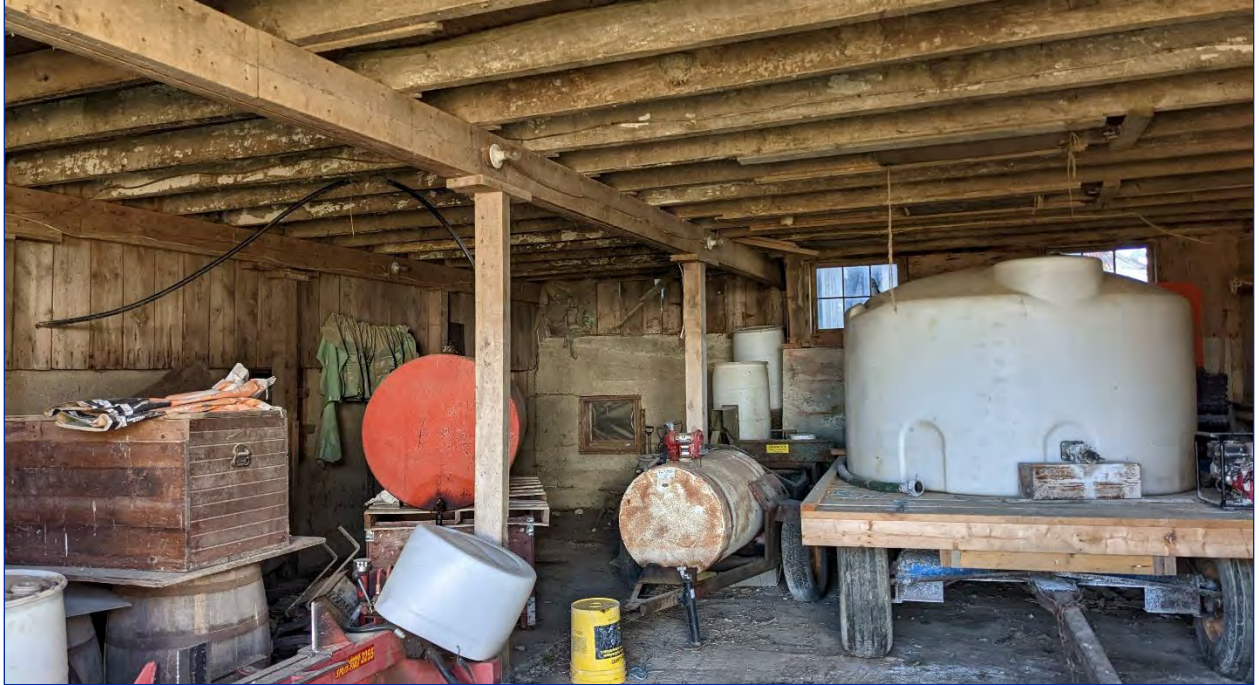
Photo 22: View of the interior of the addition on the north elevation
