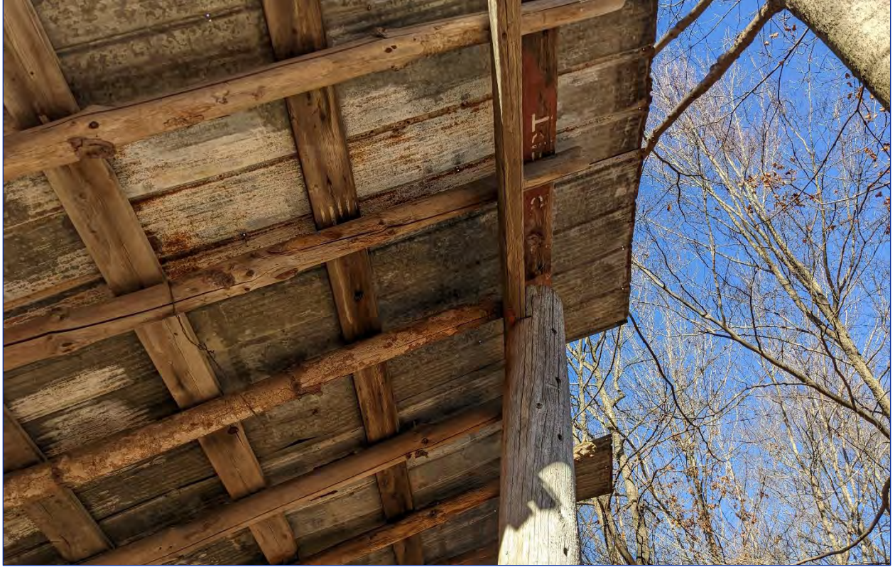
Photo 47: Detailed view of supports and metal sheeting
