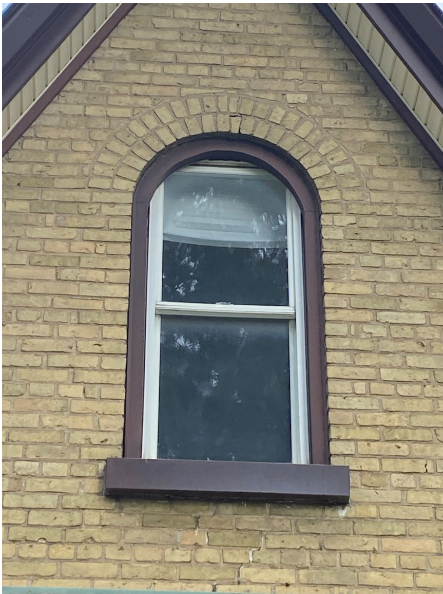
Image 8: Photograph of south facing peaked gable with double row of voussoirs over window (L. Dent, September 26, 2023)
