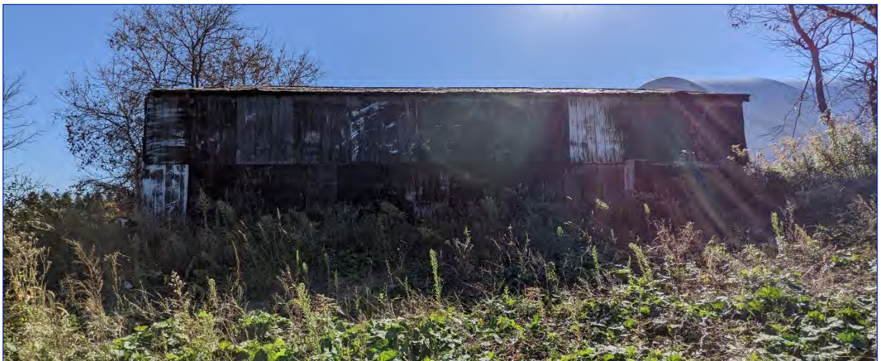
Photo 23: View of the north elevation
