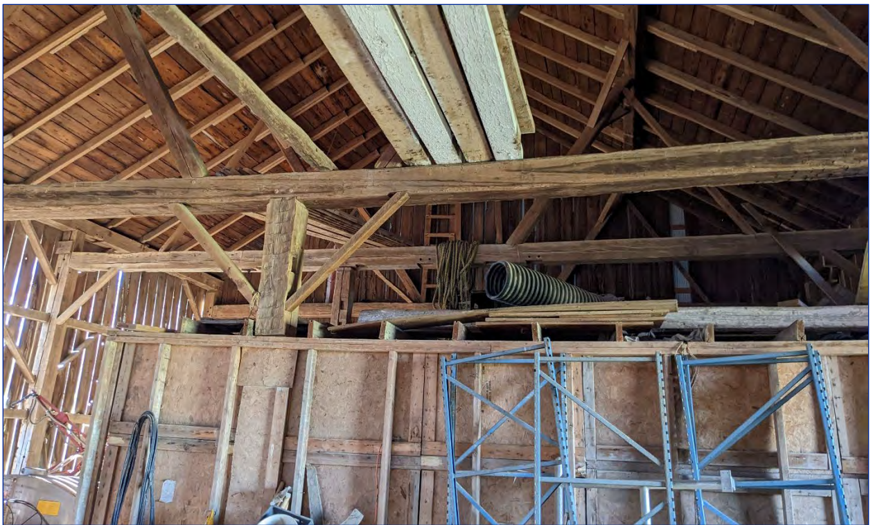
Photo 21: View west of interior
