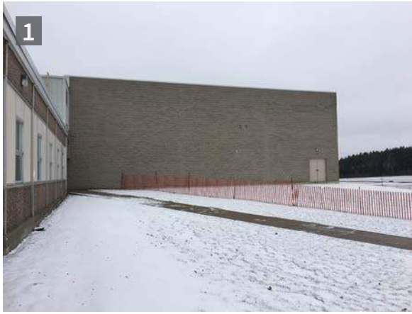
Looking north towards 1987 gymnasium addition (ERA, 2018).
