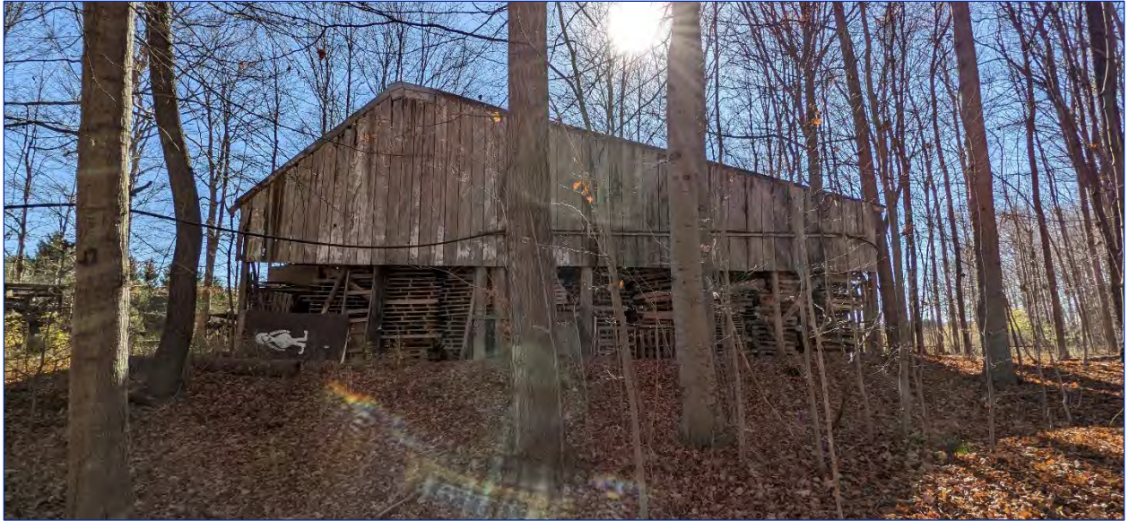
Photo 40: View of the north elevation
