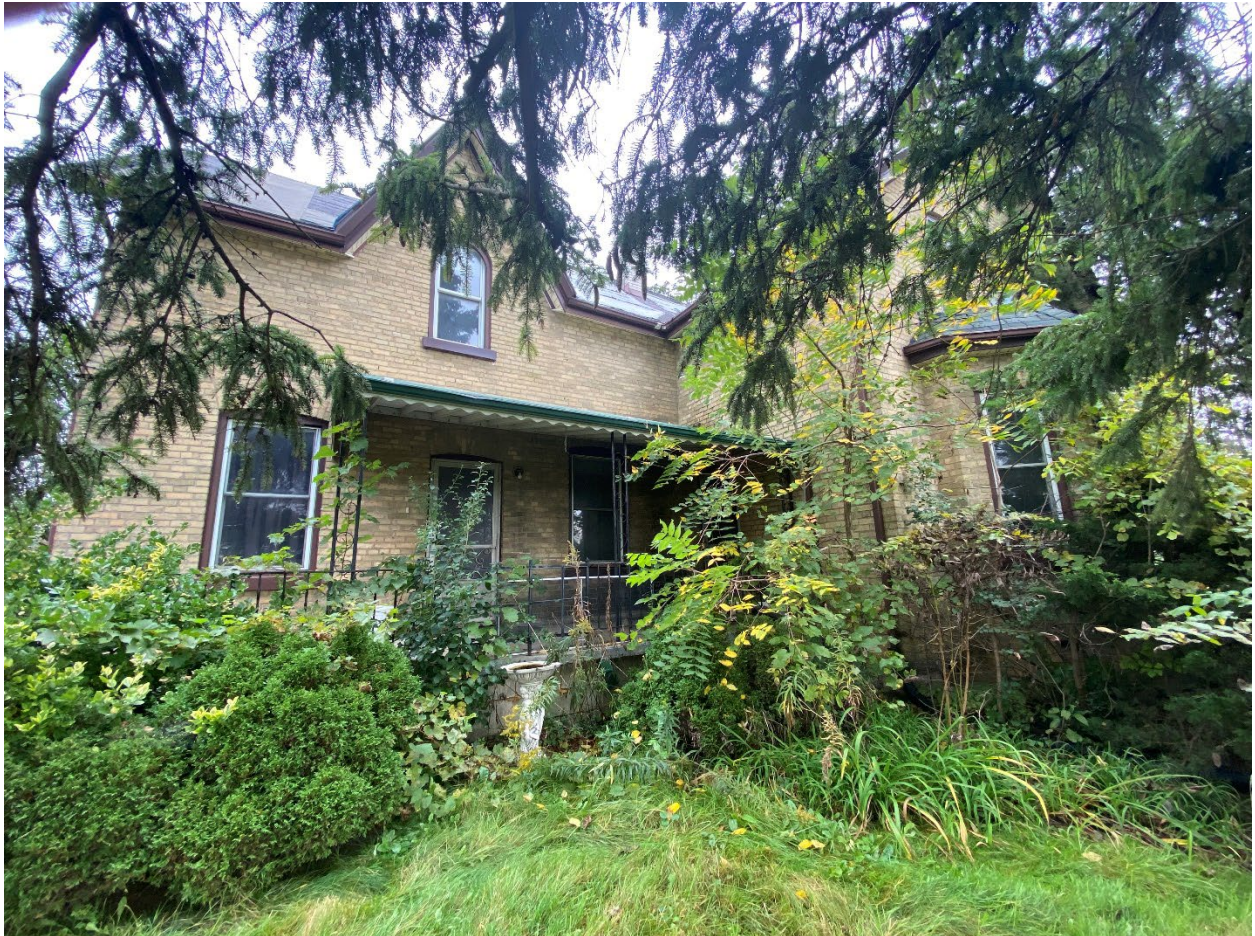
Image 7: Photograph of south facing elevation at the intersection of wing with peaked gable over entrance and gabled end with bay window (L. Dent, September 26, 2023).
