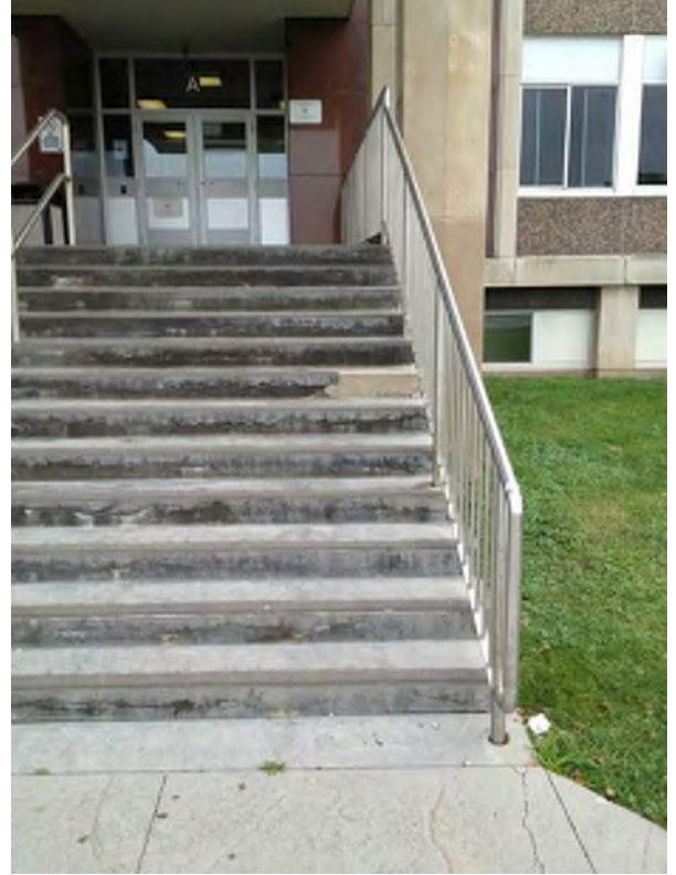
Front entry exterior stairs
