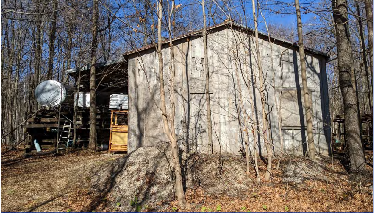
Photo 38: View of the south elevation
