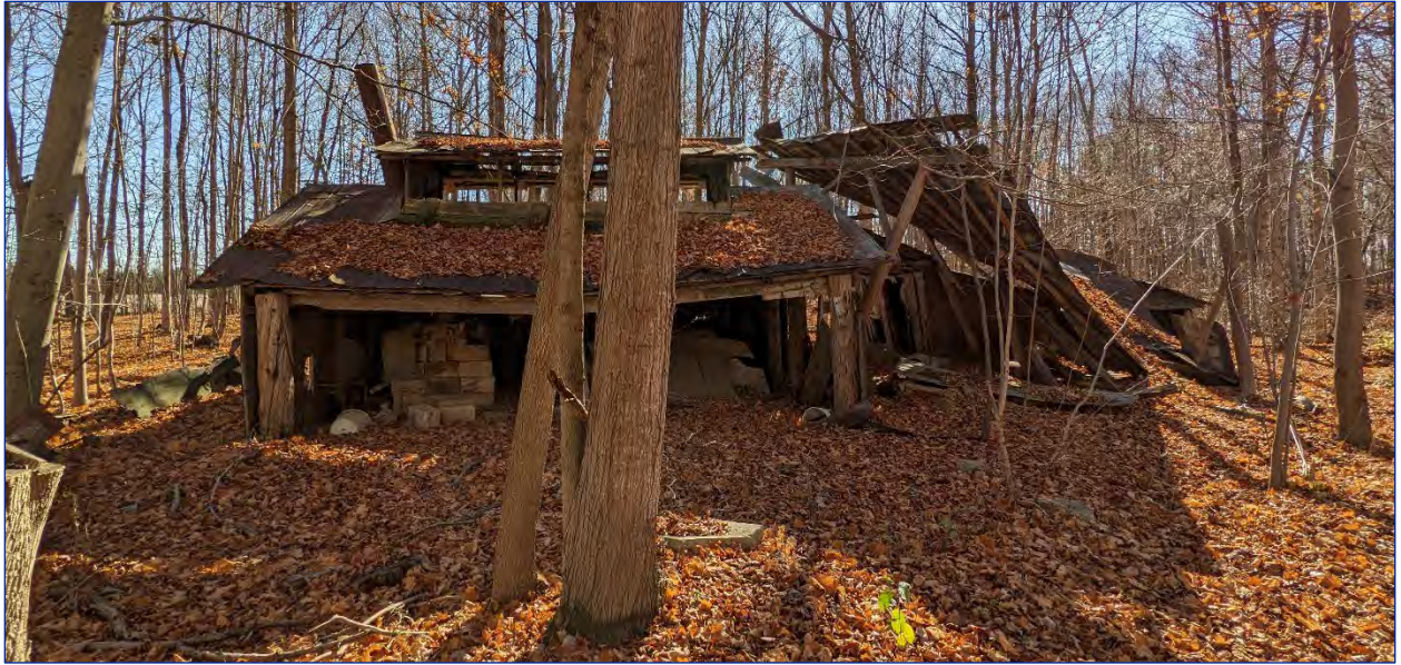
Photo 43: View of the north elevation
