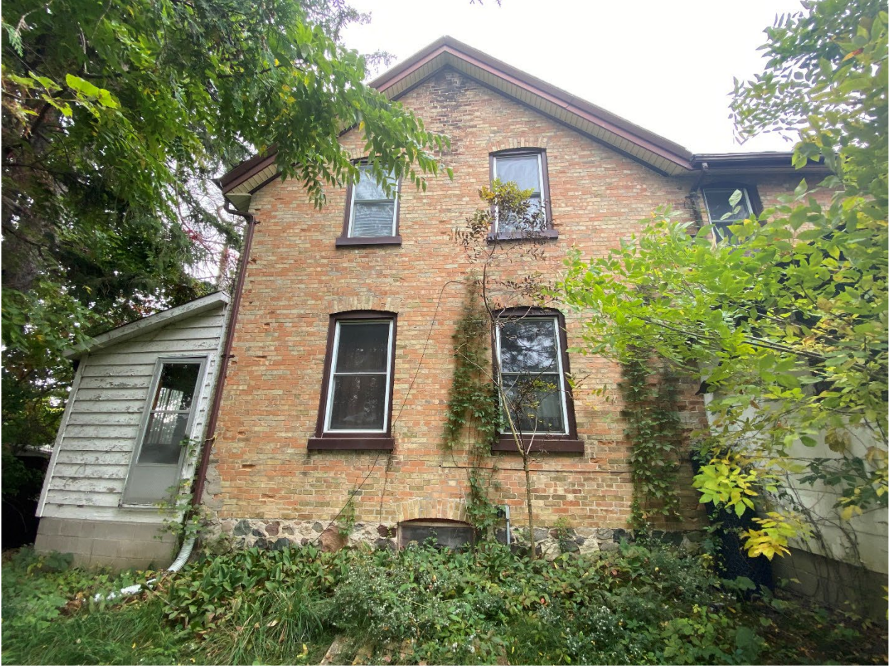
Image 4: Photograph of north facing elevation of house, close-up without projecting addition-see small addition facing east (L. Dent, September 26, 2023).
