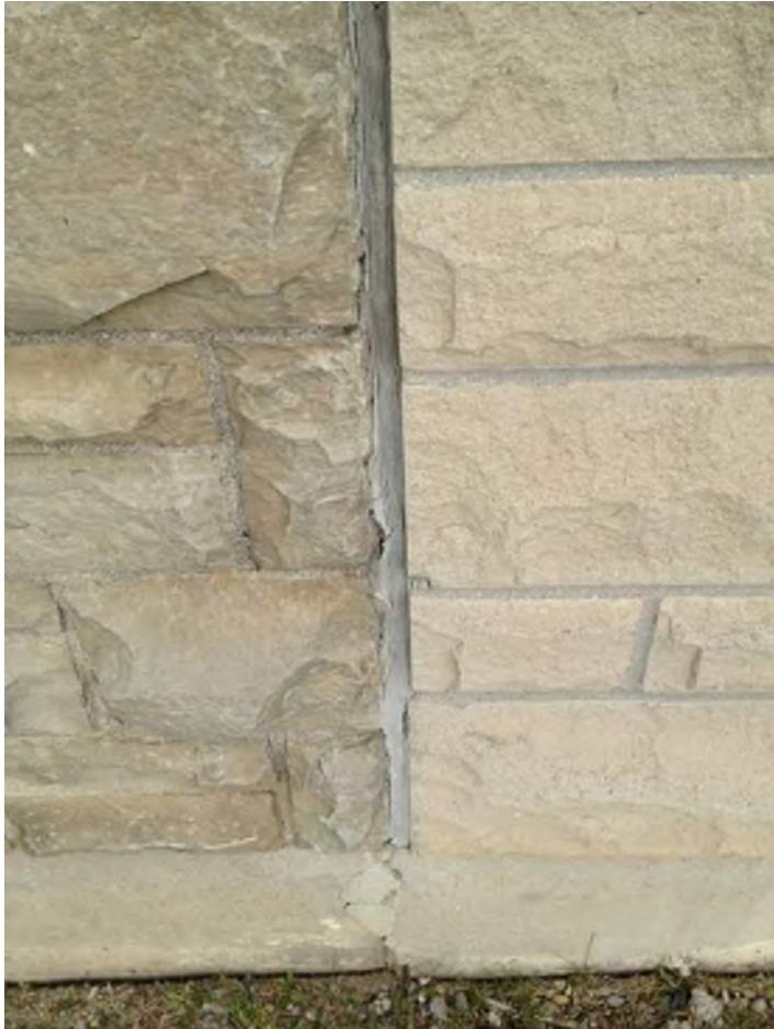
Caulked expansion joint at tech wing addition - base
