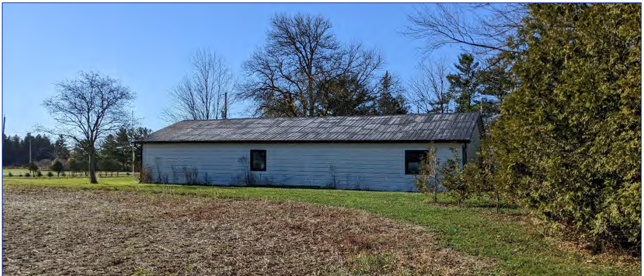
Photo 36: View of the east elevation
