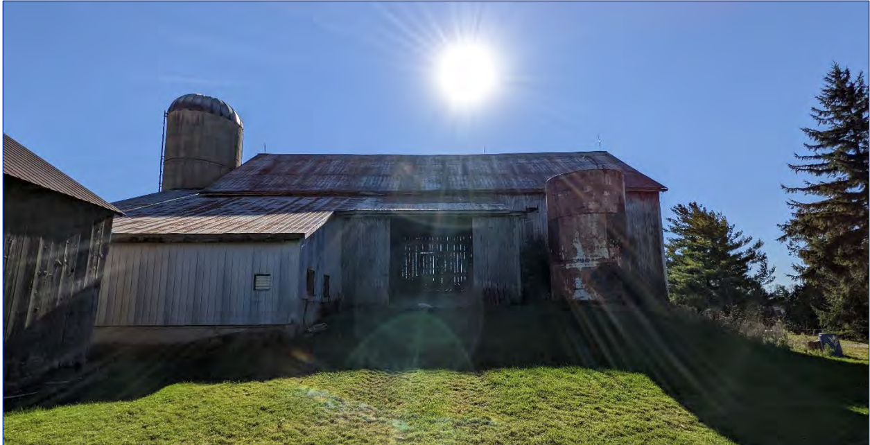
Photo 18: View of the north elevation
