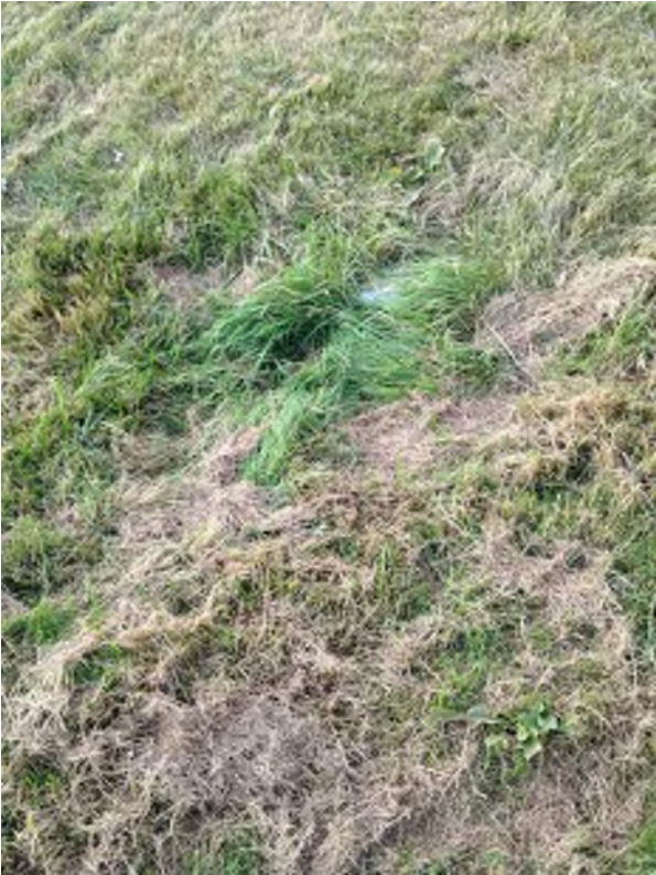
Drain culvert in grass
