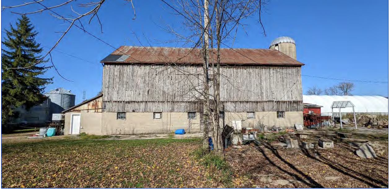
Photo 16: View of the south elevation
