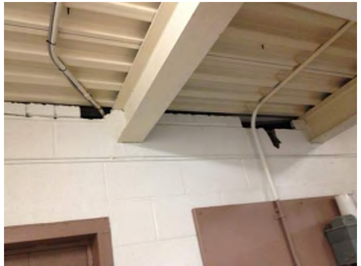
Fire separation at elevator machine room
