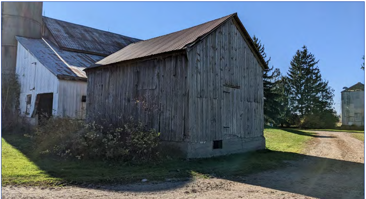
Photo 31: View of the northeast elevation
