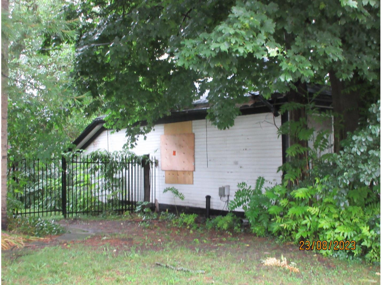
Image 4: North elevation of the building on the subject property at 176 Piccadilly Street, May 2, 2022.
