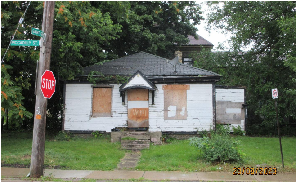
Image 1: South elevation of the building on the subject property at 176 Piccadilly Street, May 2, 2022.
