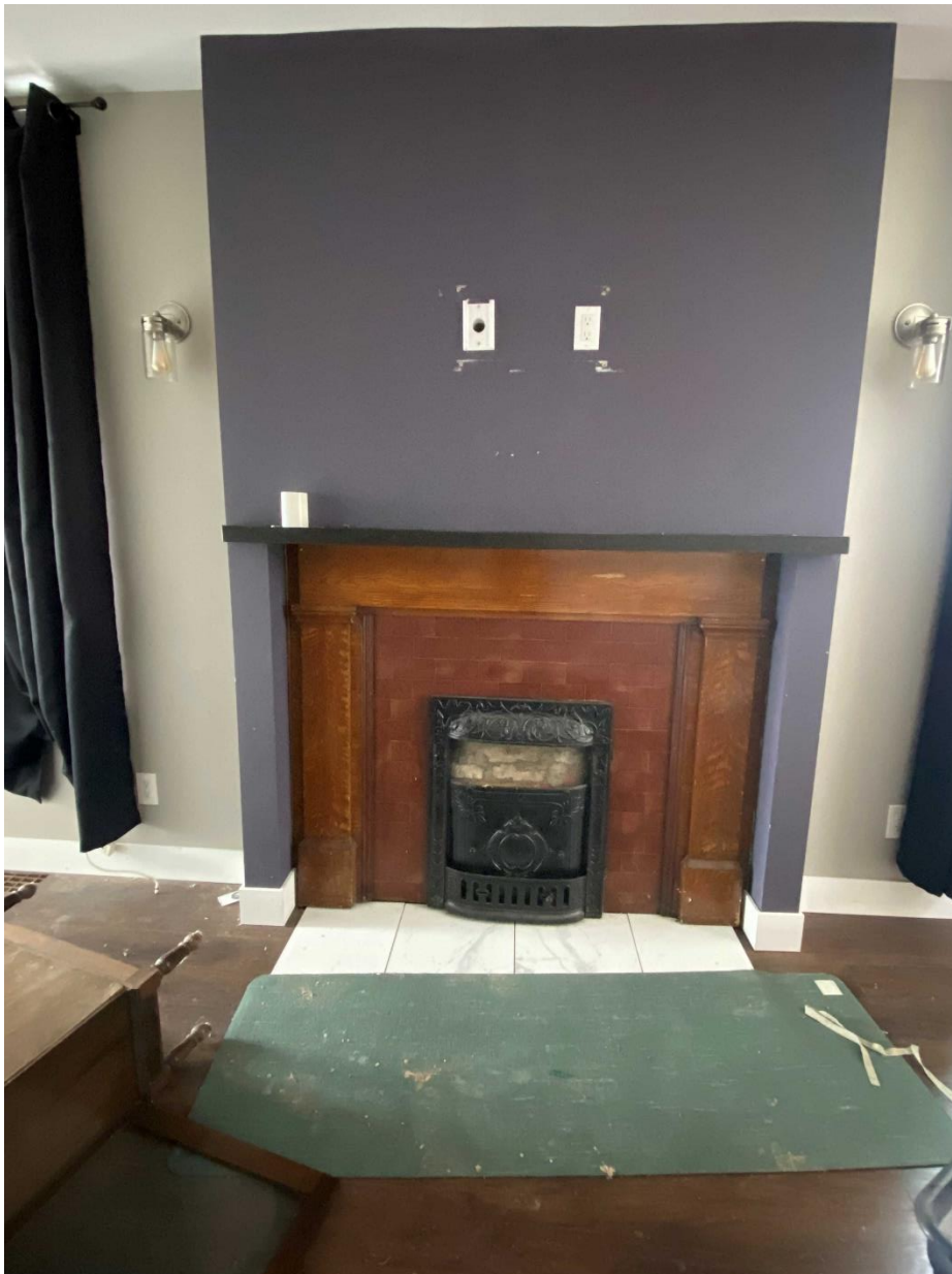
Image 13: Photograph of fireplace with insert and wooden mantel (L.Dent, March 14, 2022).
