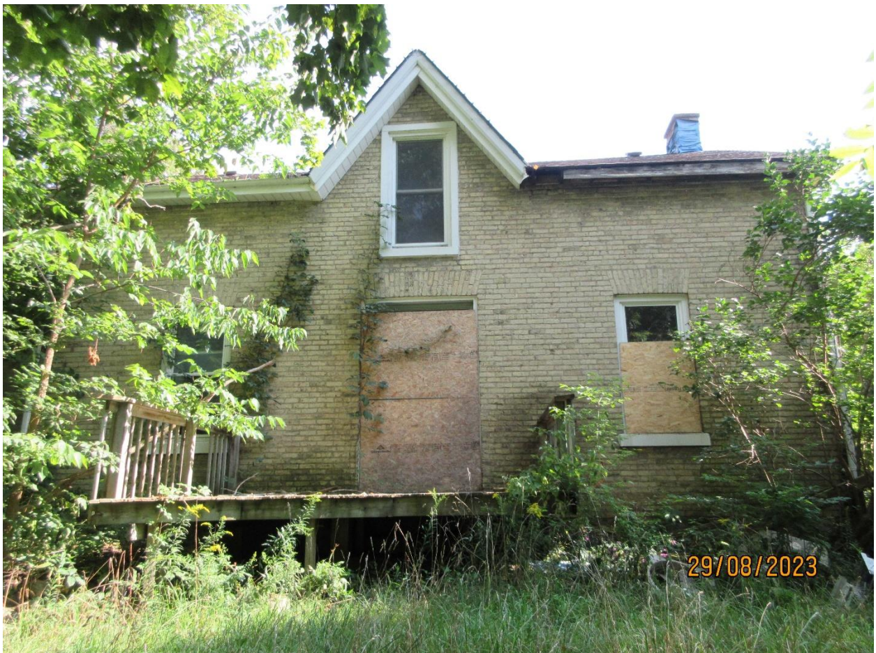
Image 7: Photograph showing north elevation of farmhouse noting flat arch brick lintels located above the window and door opening as well as vinyl window in gable (L.Dent, August 29, 2023).
