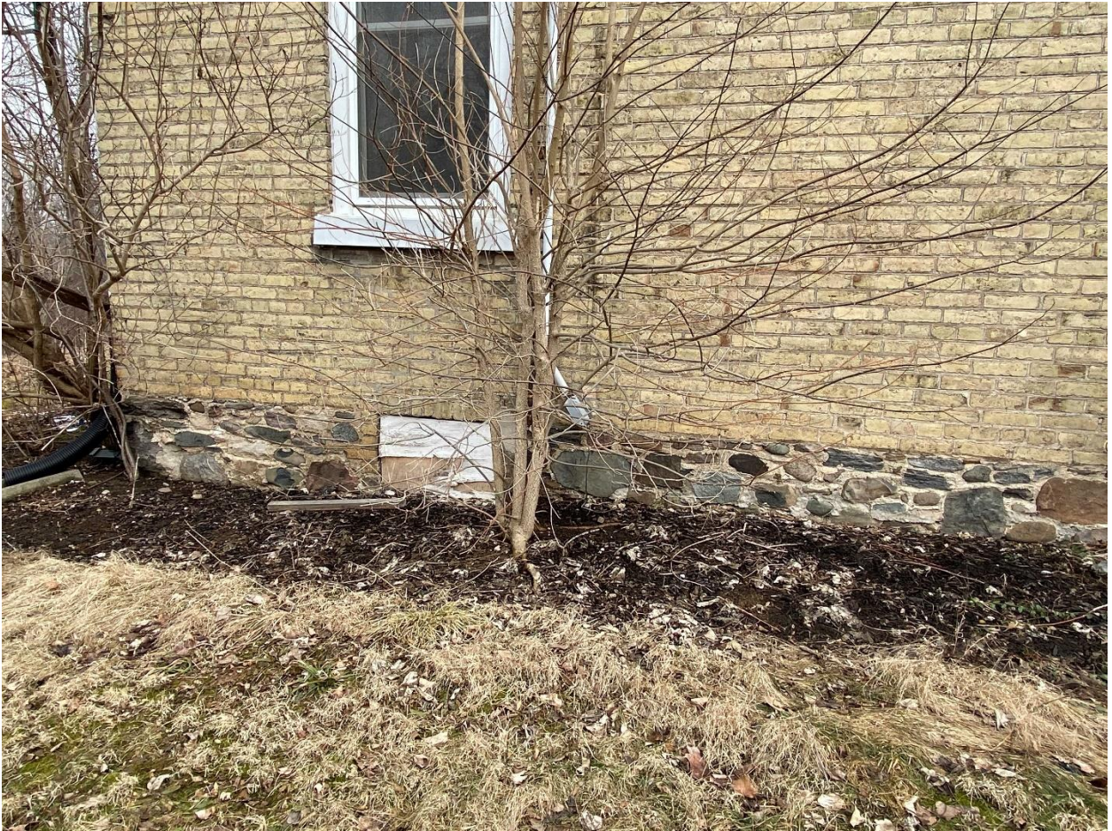
Image 8: Photograph showing stone foundation – west elevation (L.Dent, March 14, 2022).
