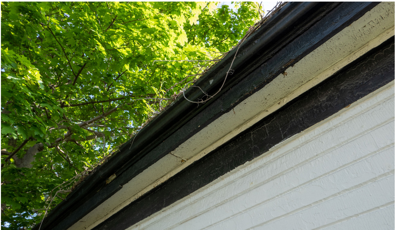
Figure 16: Detail of white soffit and black fascia boards as seen on the west elevation (CBCollective, 2023).
