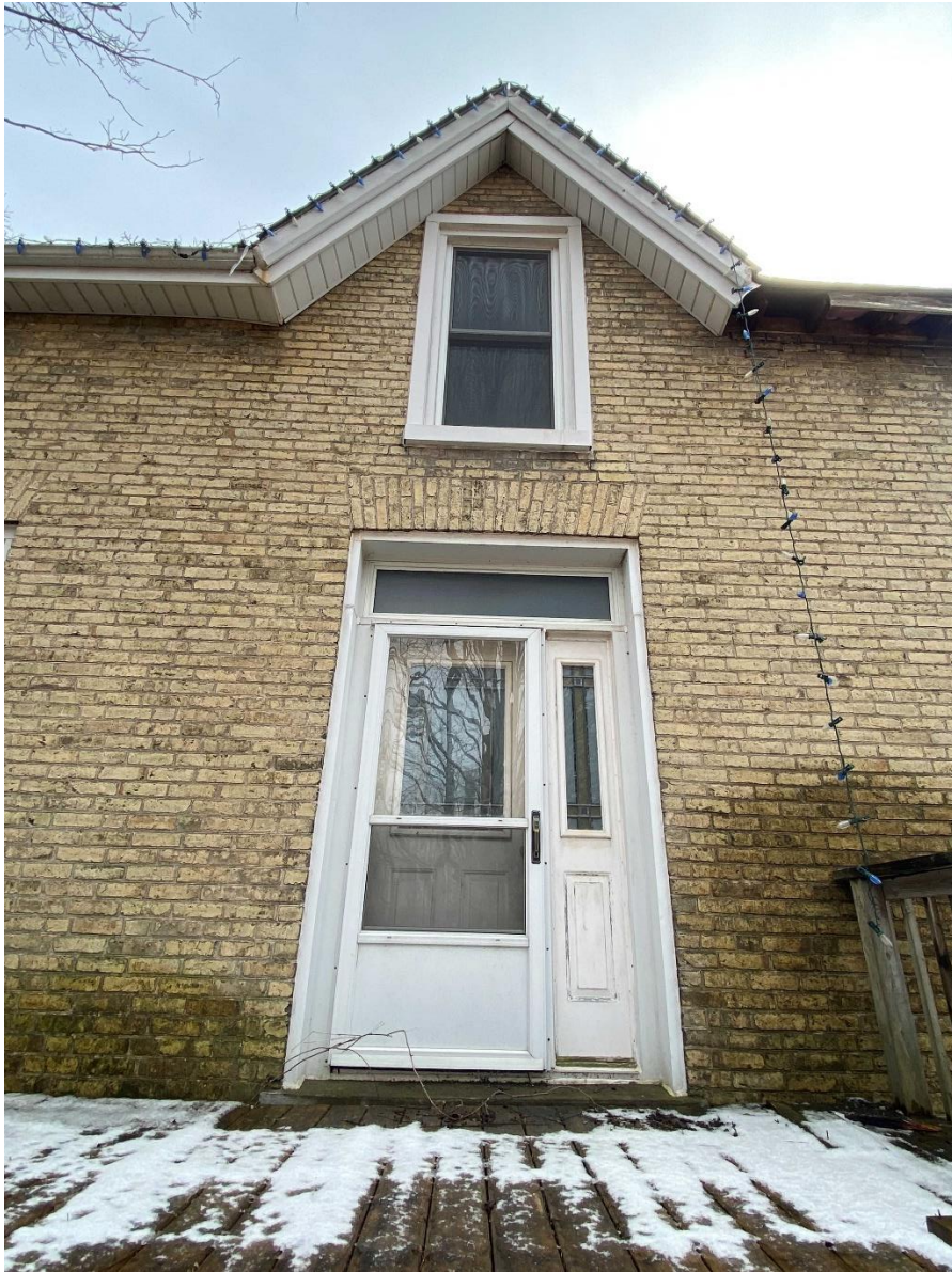
Image 6: Photograph showing entrance door with sidelight and transom prior to being boarded up – north elevation (L.Dent, March 14, 2022).
