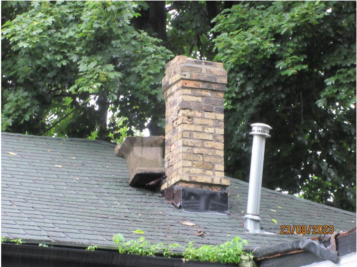
Image 7: Buff brick chimney on the east side of the building on the subject property at 176 Piccadilly Street, August 23, 2023.
