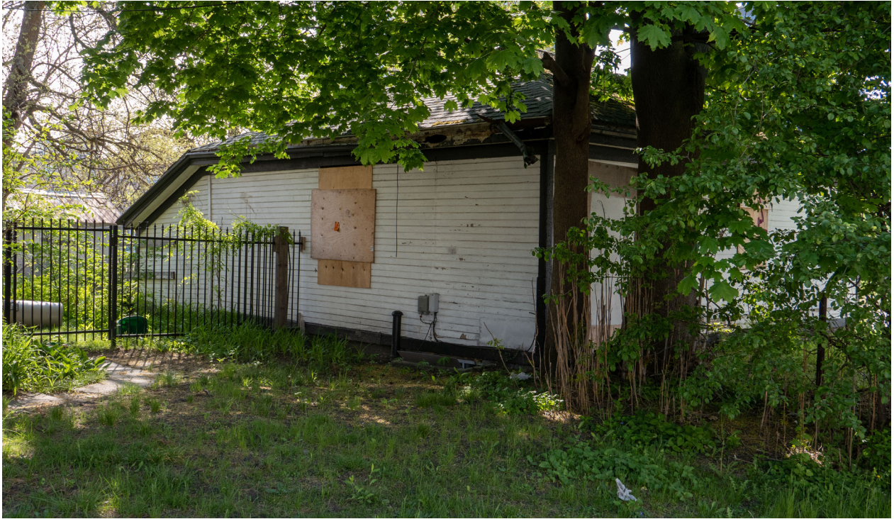
Figure 13: Configuration of the rear, north elevation (CBCollective, 2023).
