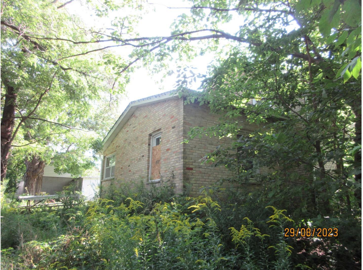
Image 9: Photograph showing addition at northeast corner of farmhouse (L.Dent, August 29, 2023).
