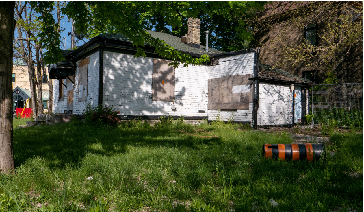
Figure 10: View of the dwelling's east elevation and east addition (CBCollective, 2023).
