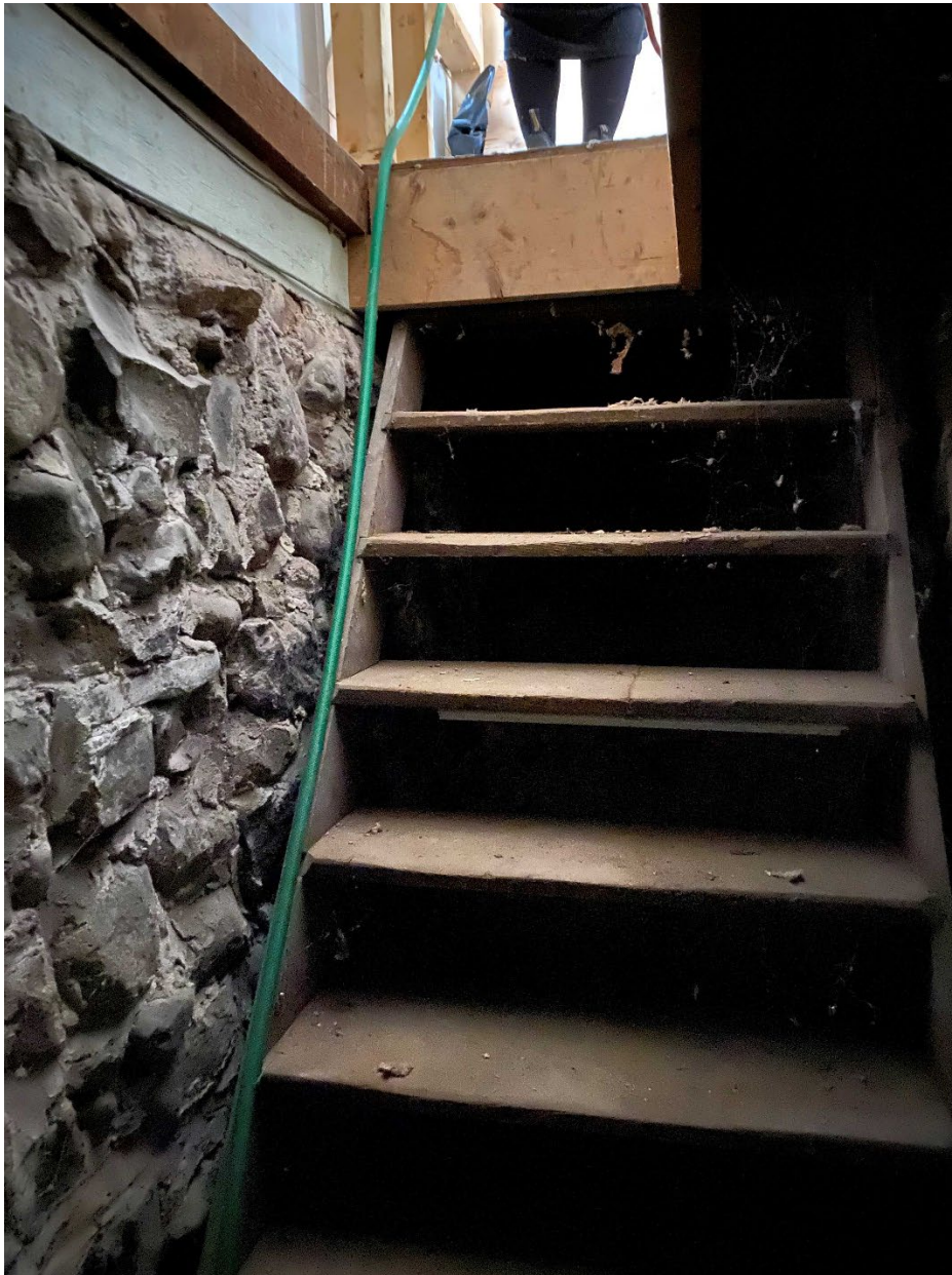
Image 14: Photograph of basement access showing stone foundation wall (L.Dent, March 14, 2022).
