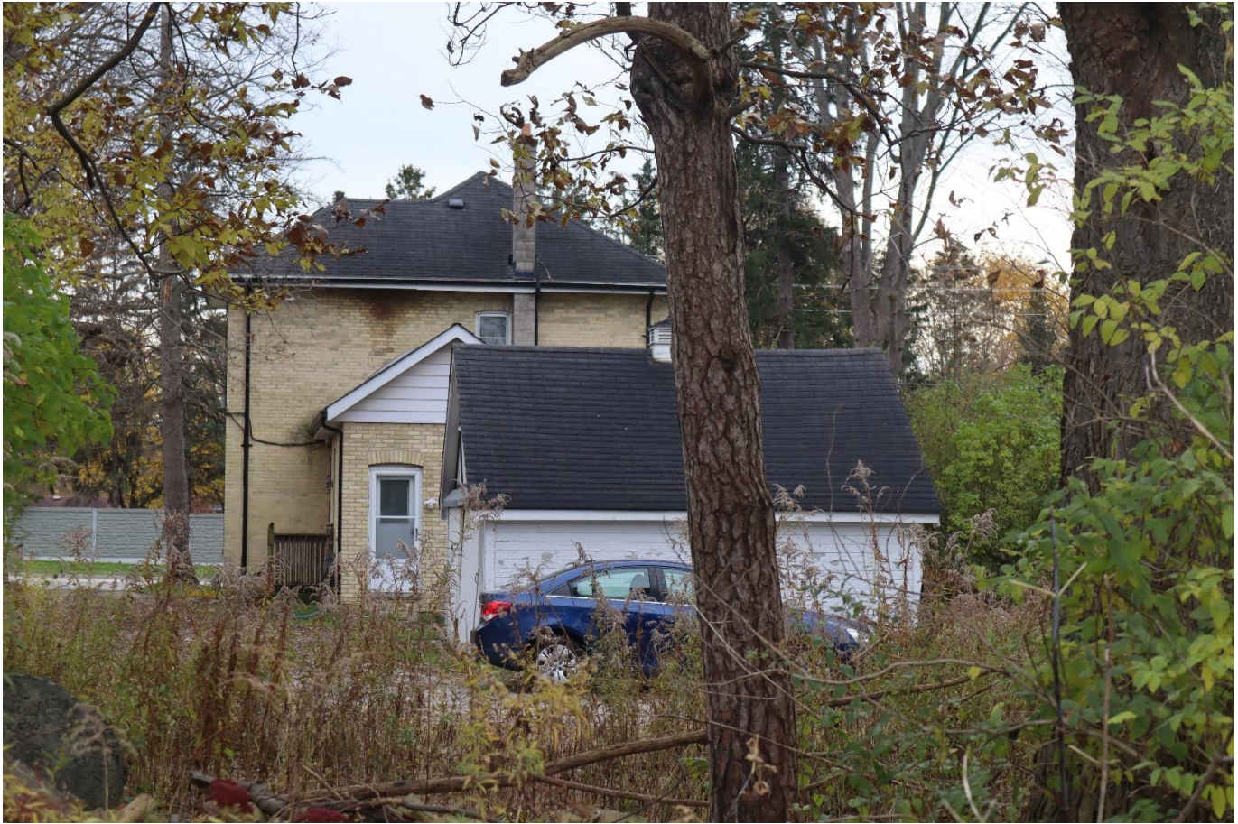
Photograph 17: View of the northern elevation, looking south (AECOM 2021)
