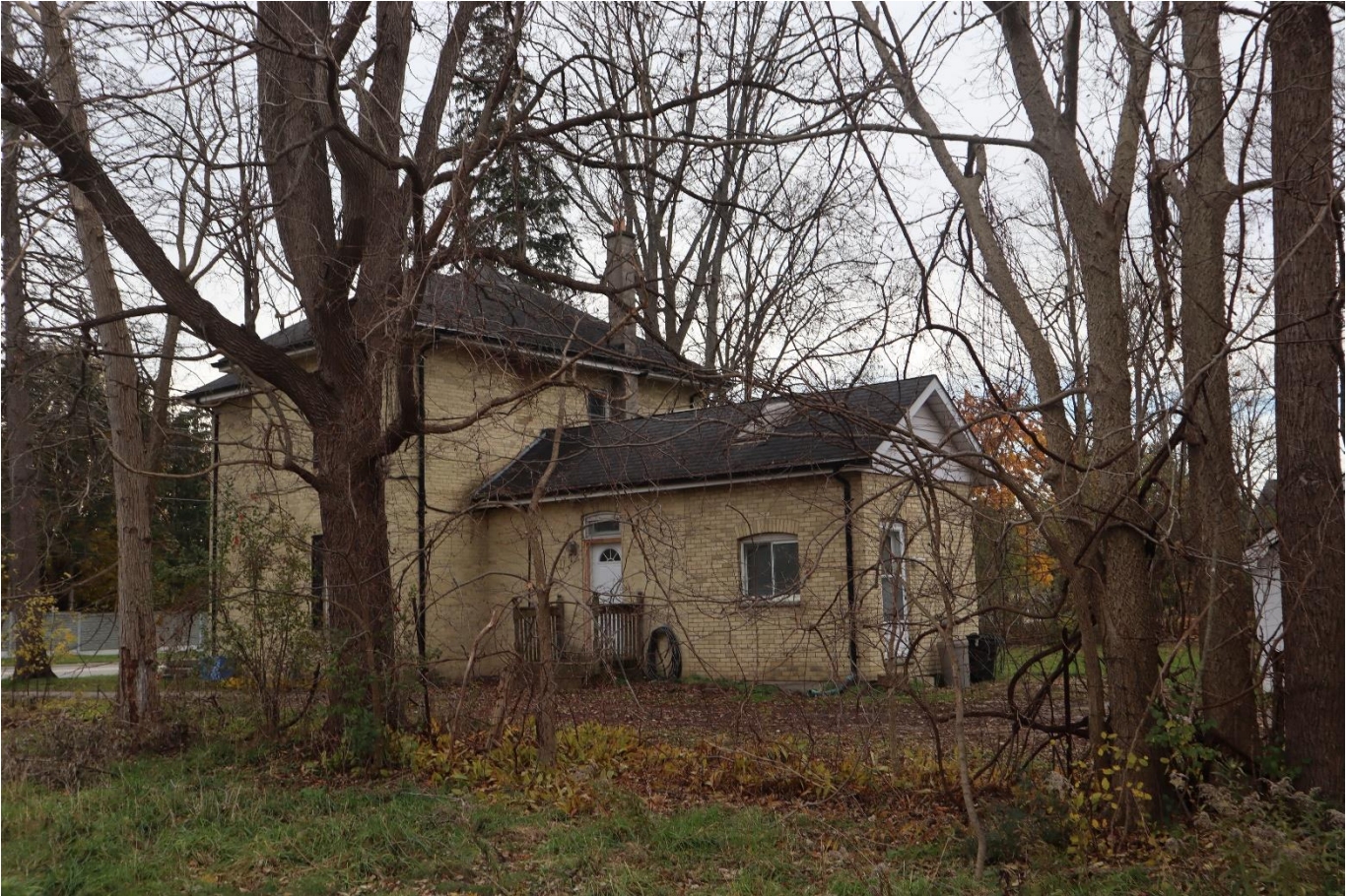
Photograph 10: View of the two-storey buck brick detached house, including the kitchen tail and rear addition located within the Study Area, looking southwest (AECOM 2021)
