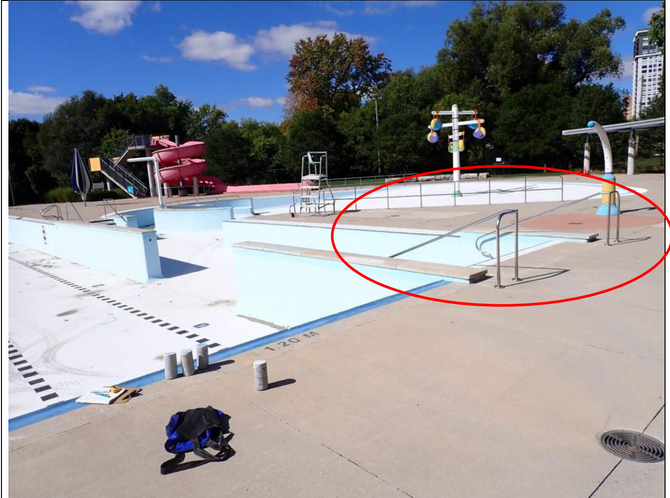
PHOTOGRAPH 5: Stainless Steel railing appears sound
