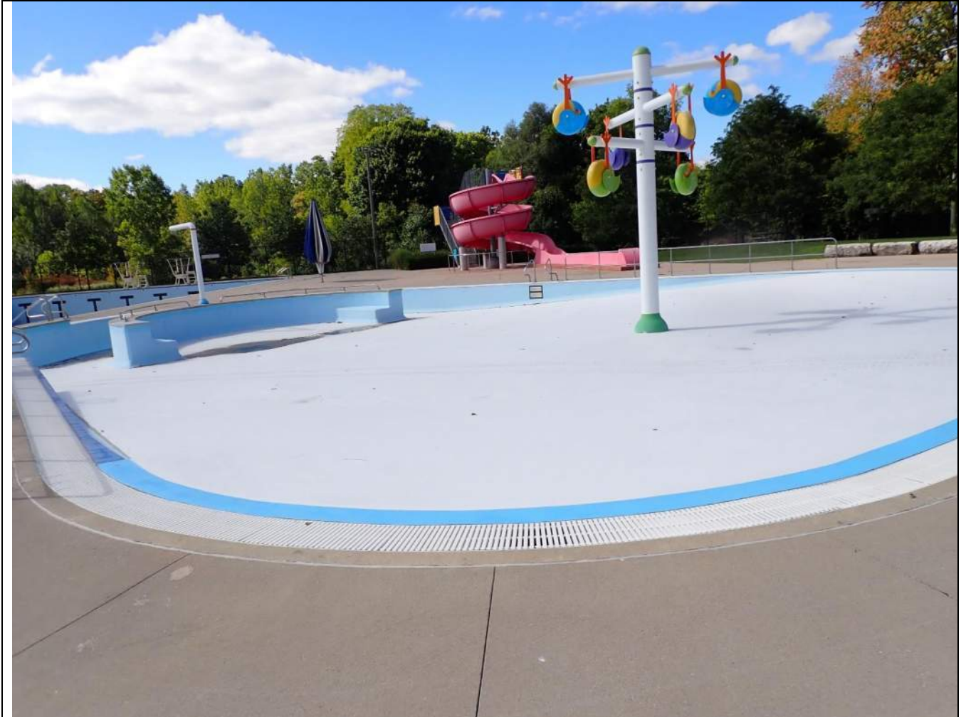
PHOTOGRAPH 3: Overview of Leisure Pool
