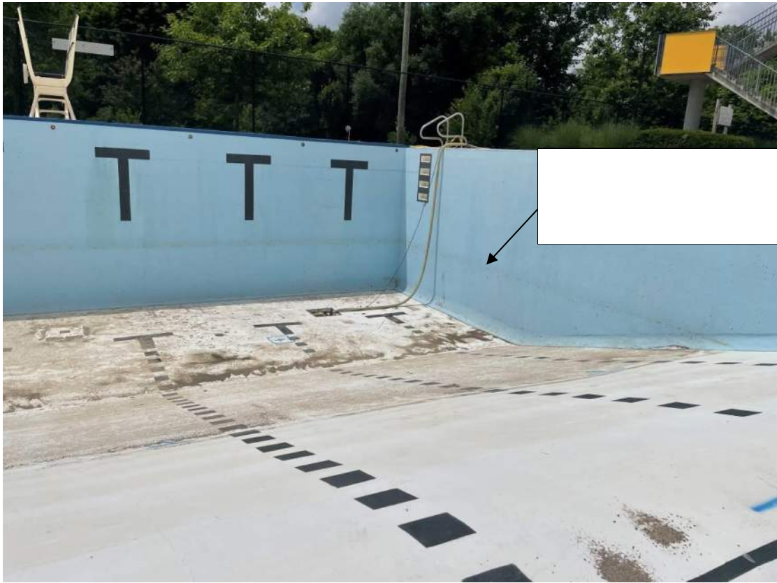
Figure 4 – Debris marking water lost line, and pump extracting ground water
