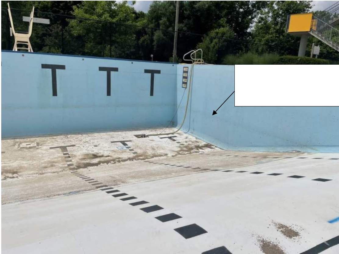
Figure 3a – Debris marking water lost line, and pump extracting ground water (June 2022)
