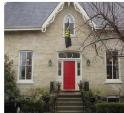
7. Italianate-influenced segmental arches of the windows and entranceway
