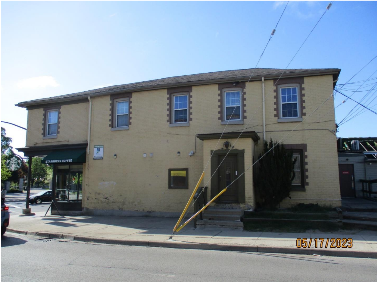
Image 9: Photograph showing north facade of the building at 601 Richmond Street, fronting onto Central Avenue.
