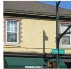
4. Row of second storey window openings, and painted brick surrounds on the east façade.
