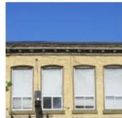
4. Symmetrical row of six arched window openings and stone sills on the second storey of the east façade.
