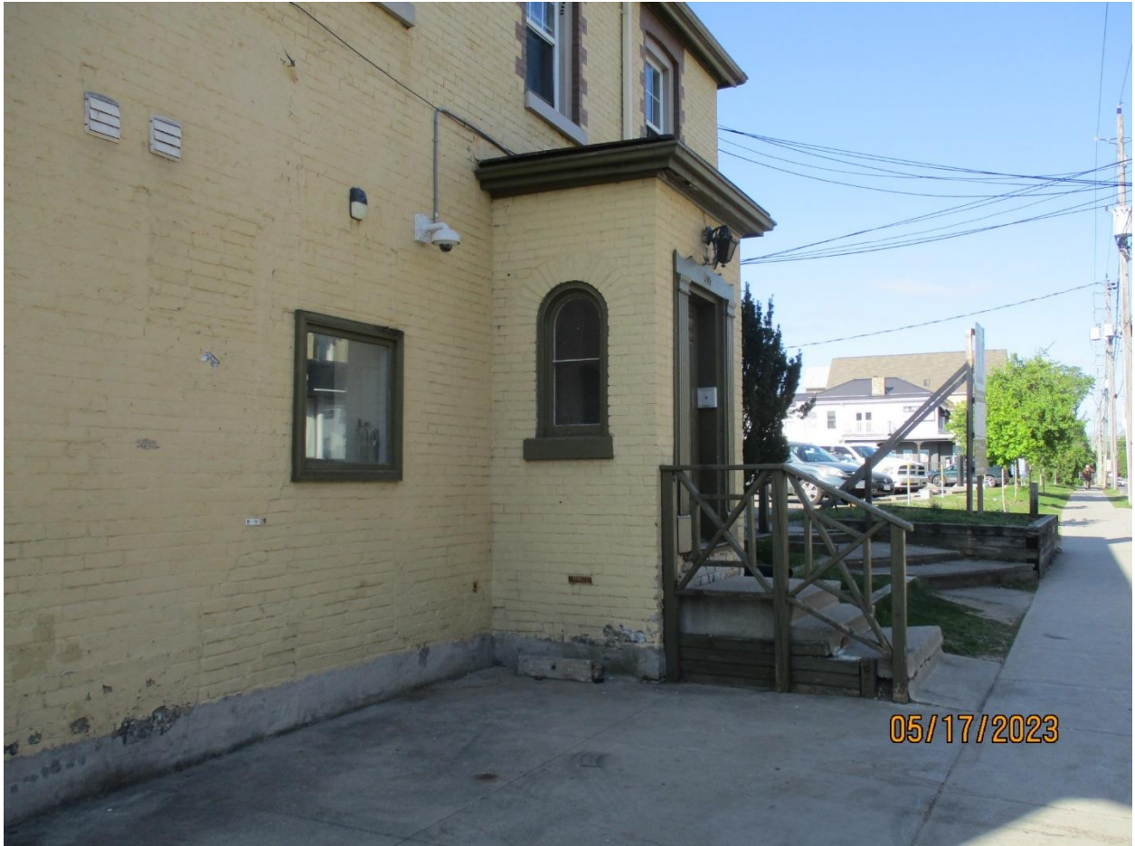
Image 11: Photograph showing side (north) entry to building at 601 Richmond Street.
