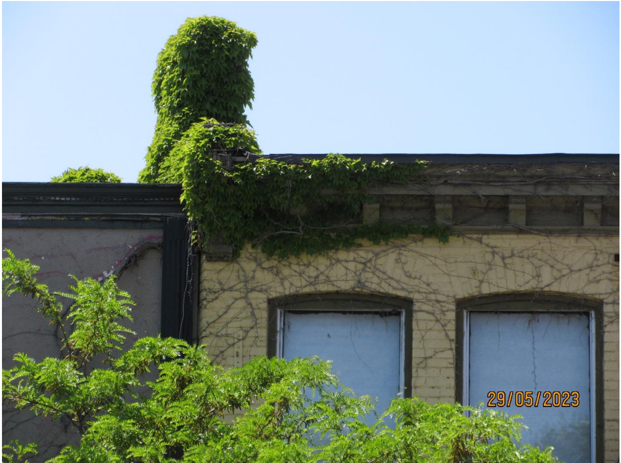
Image 5: Photograph showing roofline, cornice, corbel, and bracket details on the building at 599 Richmond Street.
