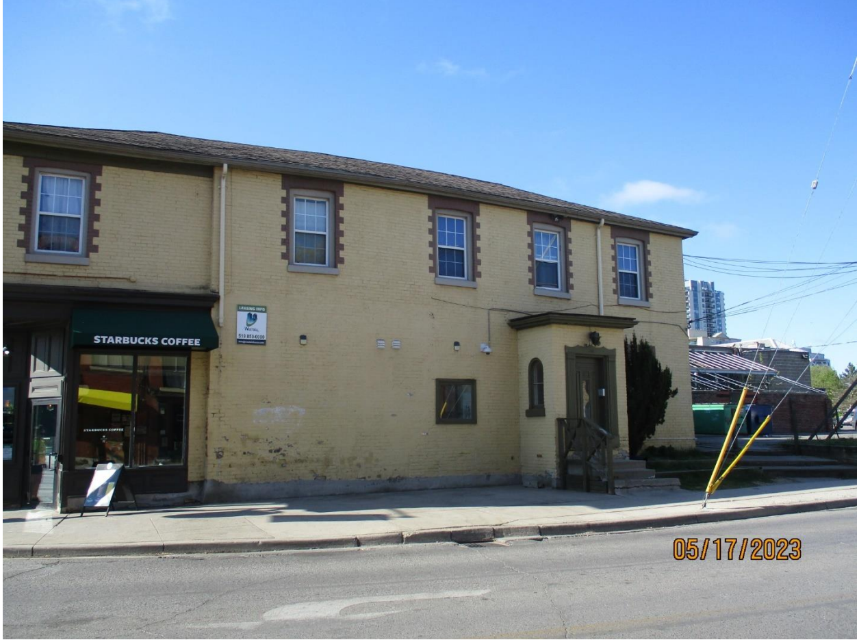
Image 10: Photograph showing north facade of the building at 601 Richmond Street, fronting onto Central Avenue.
