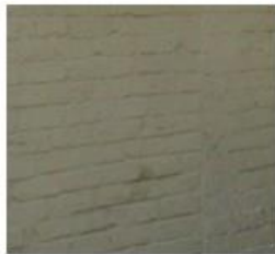
2. Painted brick veneer exterior on the east and north façades of the building.
