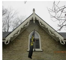
6. Replicated bargeboard, finial and drop in the front cross gable
