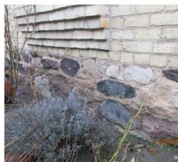
11. Fieldstone foundation walls
