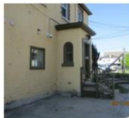
5. Projecting enclosed entry vestibule on the north façade including a) decorative panel door, b) decorative wood door surrounds, and c) arched window on the east and west sides of the entry vestibule.
