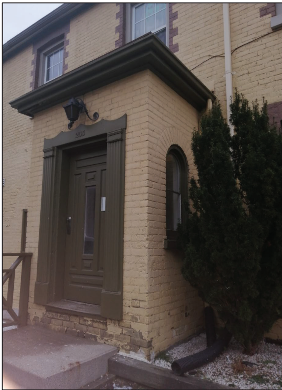
Figure 34: View of enclosed portico looking south-west (Source: MHBC, 2020).
