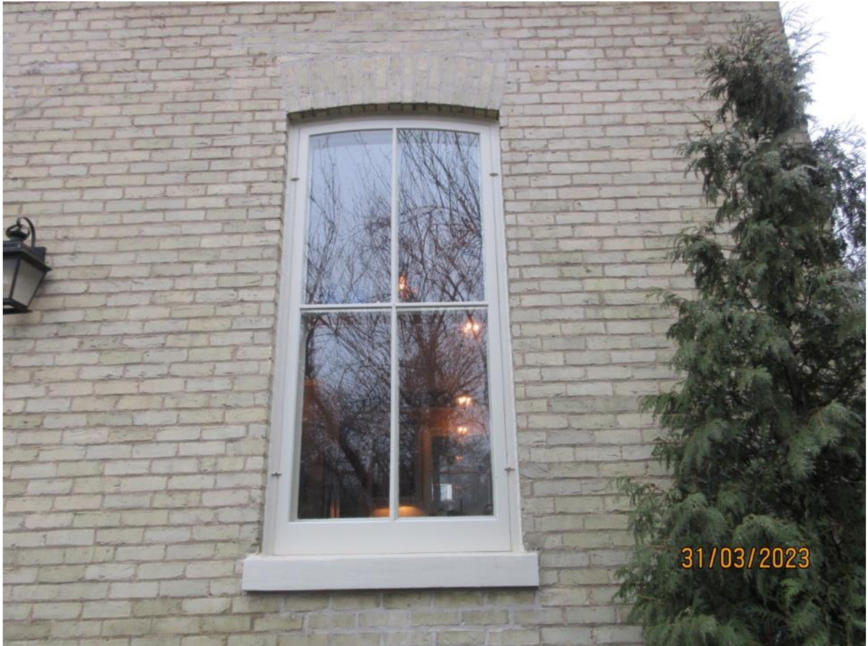
Image 3: Two-over-two wood window with wood storm window and segmental arch in the southern bay of the main (west) façade of the Alexander Leslie House at 81 Wilson Avenue.
