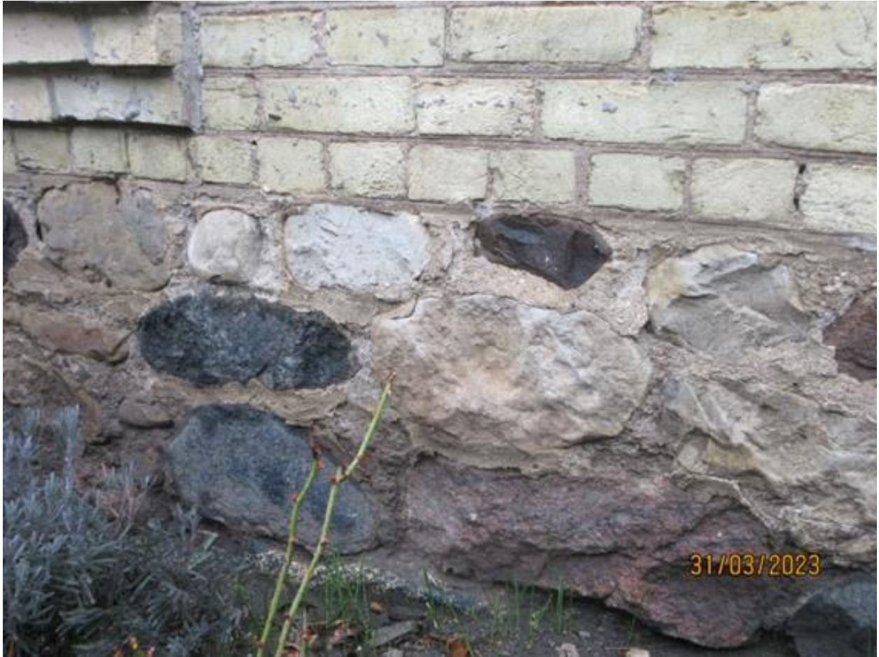
Image 9: Fieldstone foundation wall on the west elevation.
