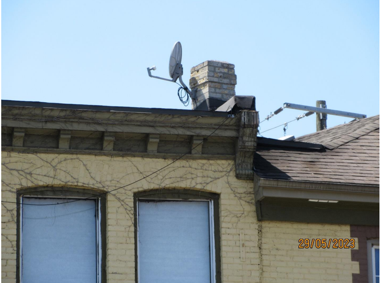
Image 4: Photograph showing roofline, cornice, corbel, and bracket details on the building at 599 Richmond Street.
