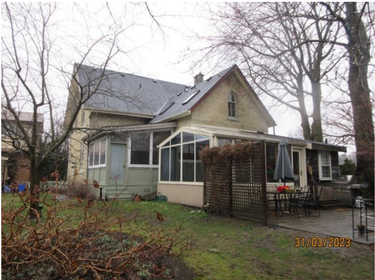
Image 6: East elevation showing back wing and T-plan of building. The side porch has been enclosed, and a conservatory has been added at the rear of the house.
