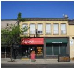
1. The form, scale, and mass of the two-storey commercial form building.
