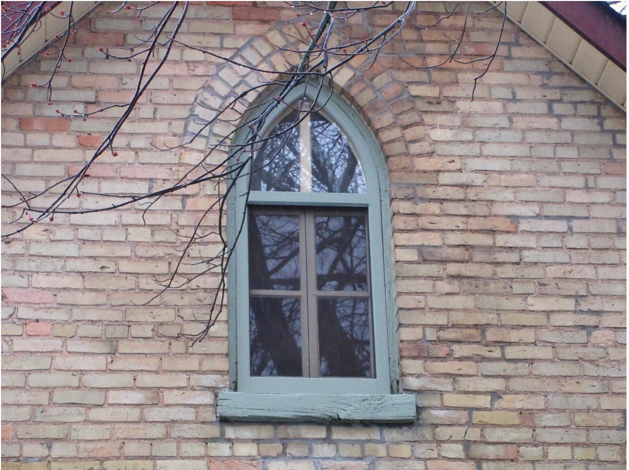
Image 7: Pointed Gothic window in the back wing.
