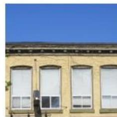
4. Symmetrical row of six arched window openings and stone sills on the second storey of the east façade.
