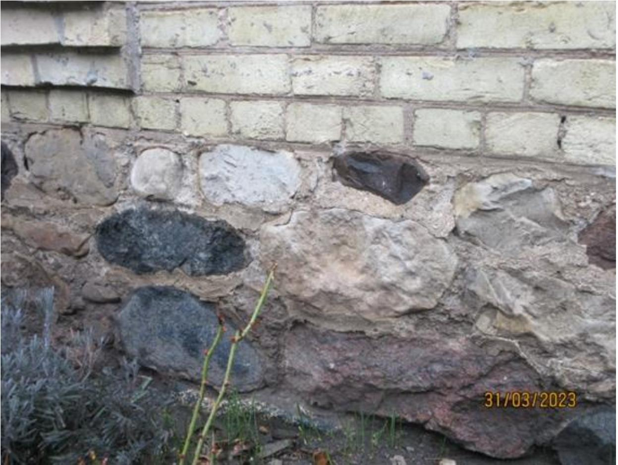
*Image 9: Fieldstone foundation wall on the west elevation.*
